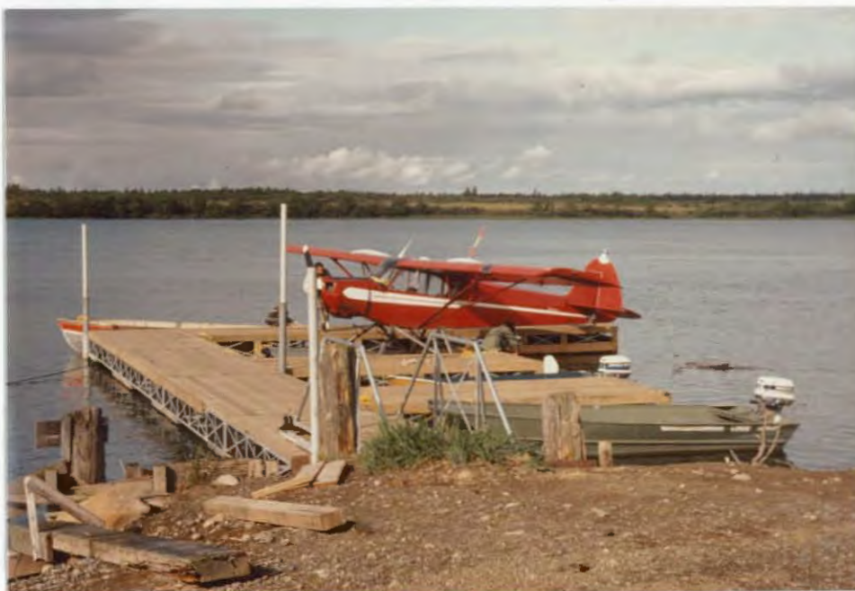
The finished product on the Naknek River. The dock rides steel pipes with the fluctuating tide. the wheeled ramp allows safe access regardless of dock height. 20-83-JT
