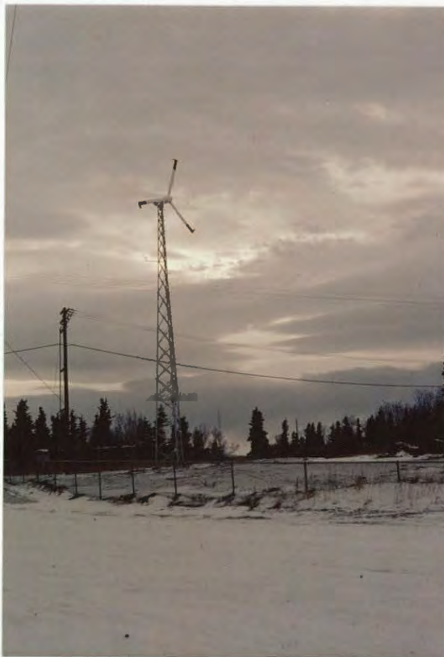
The 4.5 KW Entertech wind generator is again producing electricity for use at the refuge headquarters. 22-83-VB
