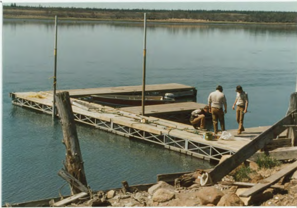
The dock purchased in 1983 is structurally sound but the design hinders quick installation and removal. CJW
