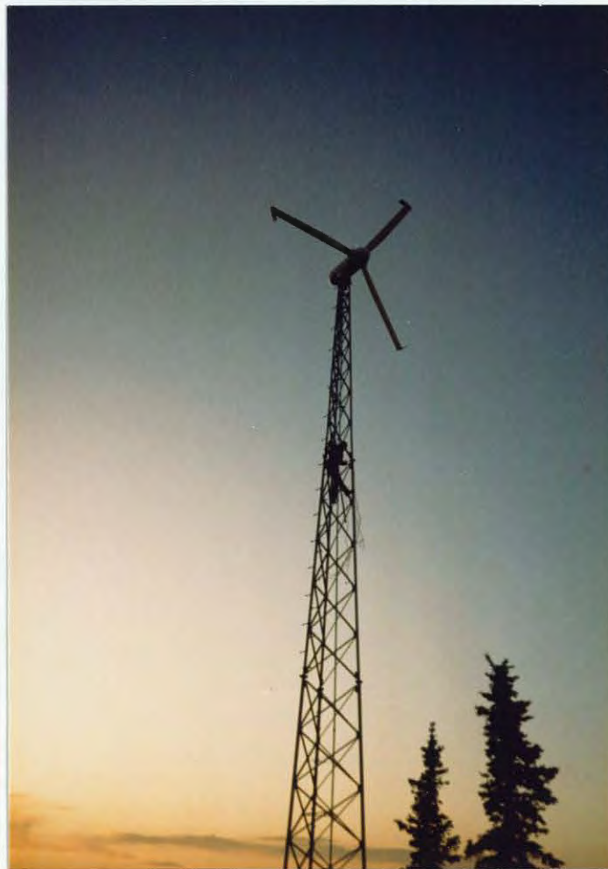
Enertech 21/5 wind generator. REH
