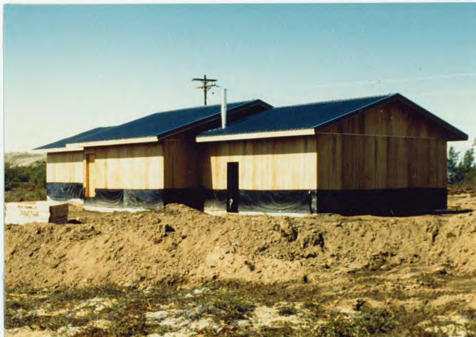
Rear view of new refuge house under construction.
