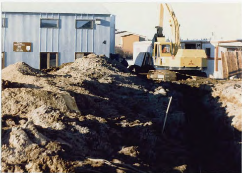
Martin Construction Company installing the new refuge water system. DDM
