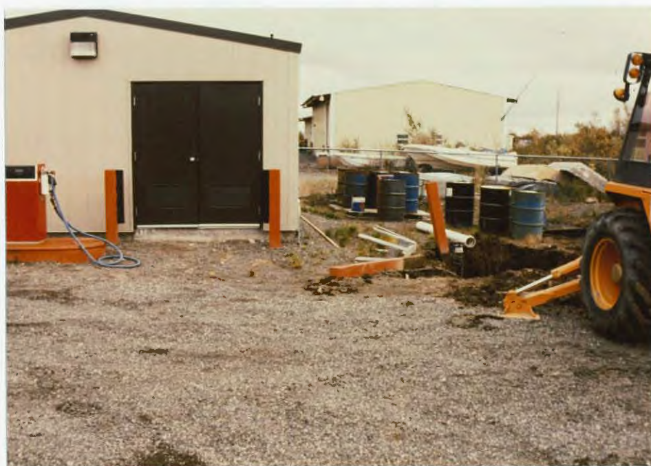
The refuge gasoline tank was filling with rainwater causing major problems with the operation of vehicles. The "no go" fuel filter was allowing water to pass thereby putting gallons of water in a vehicle's tank during a fill-up.
