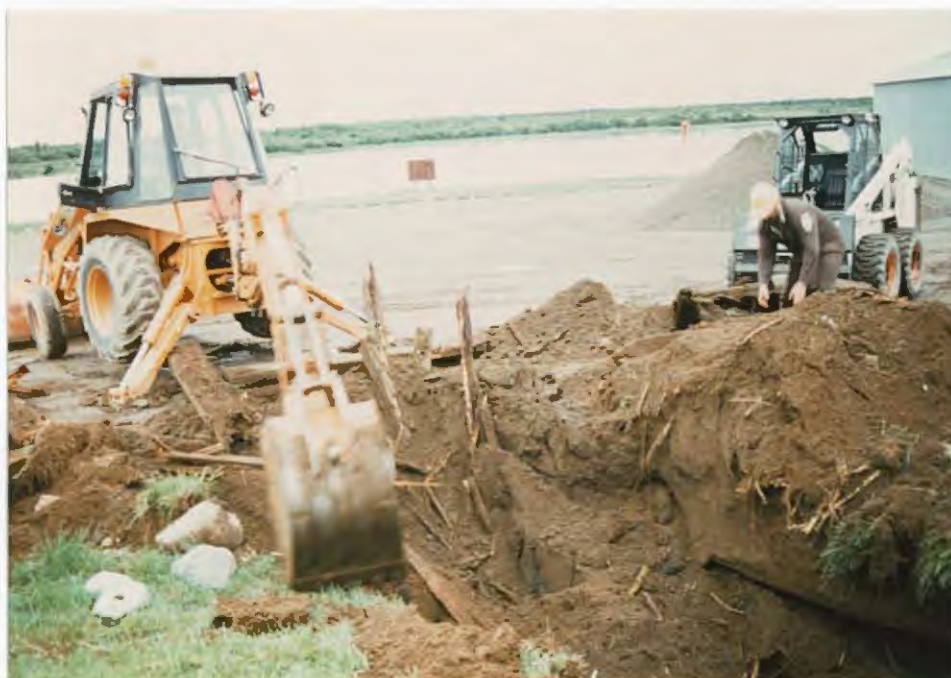
MW Terry and MH Mumma working on removing 1939 wooden septic crib. 08/03/92, REH
