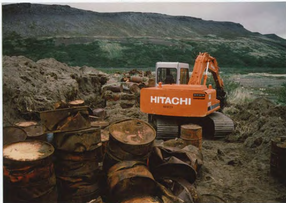
Extracting the 55-gallon barrels from the cache soon revealed a contaminants problem. 6/15/92, REH
