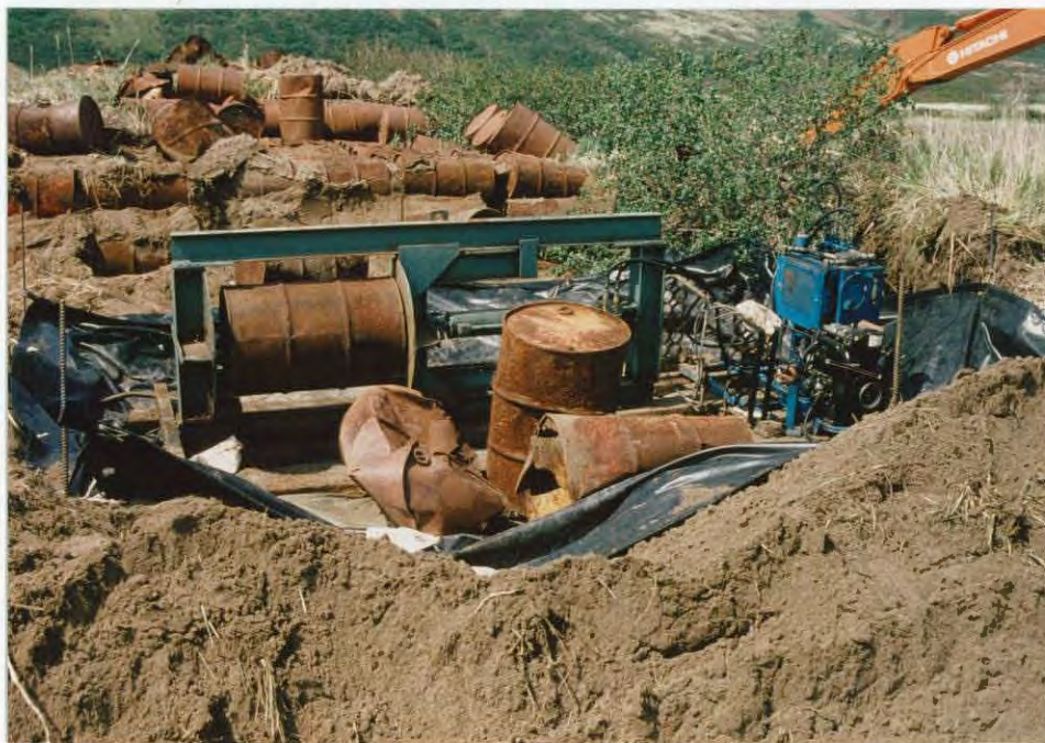
Crushing the barrels created an additional potential problem when residual fuels were discovered in many of the barrels. 6/14/92, REH
