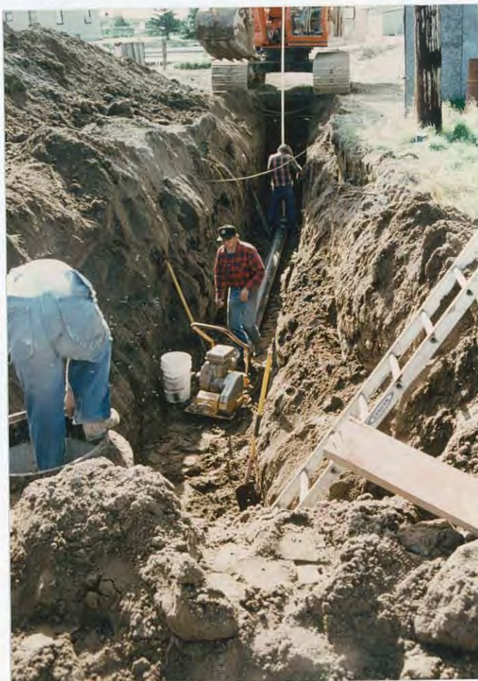
Contractors for the Borough working amongst the "whitesox" (biting bugs) to install the new sewer piping system. 07/92, REH
