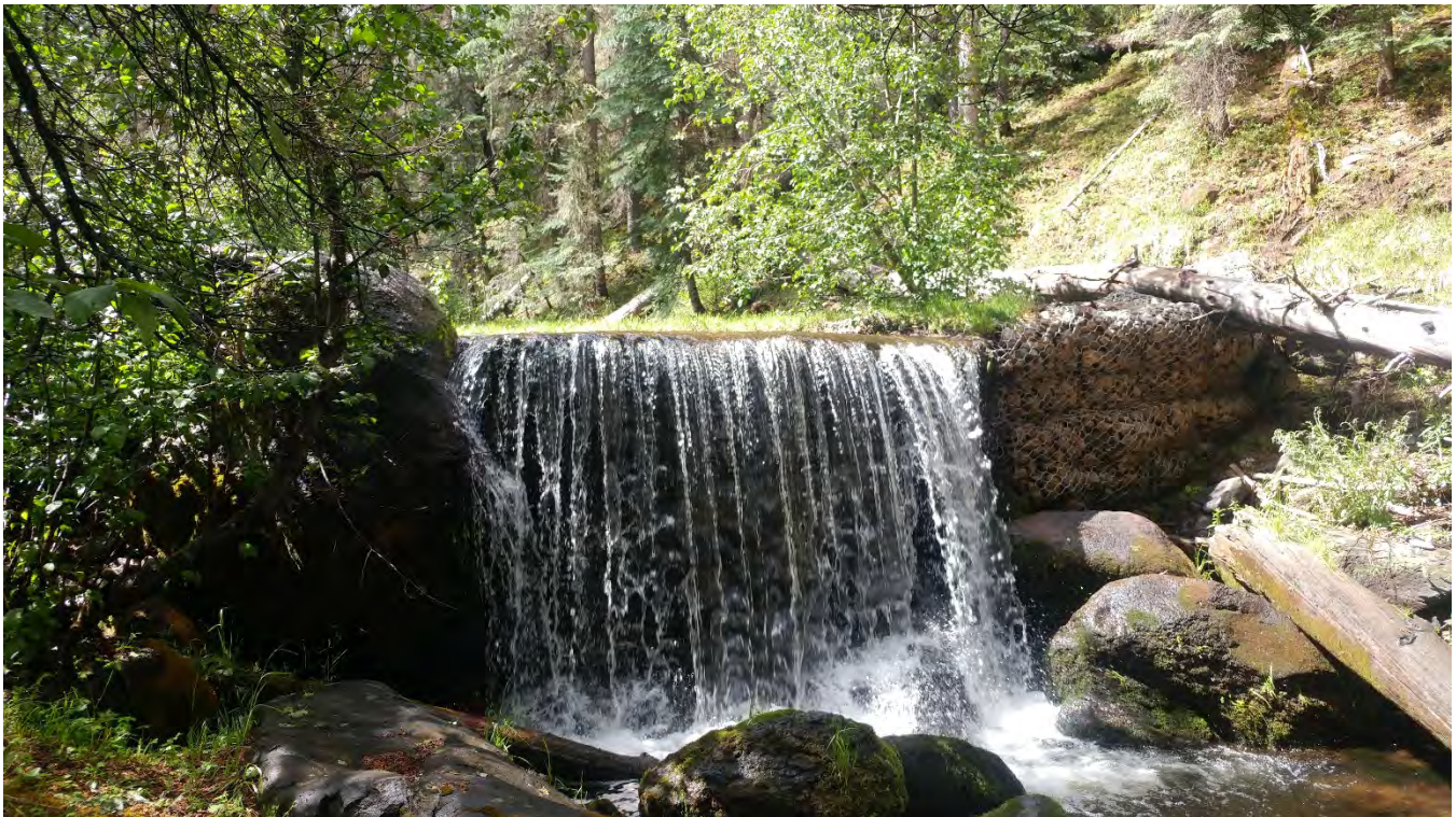
Protective gabion barrier on Paradise Creek, Arizona.
