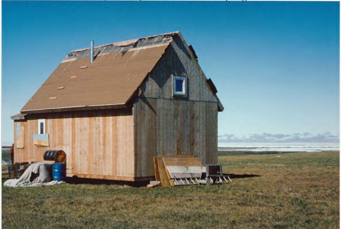
This survival shelter, placed on an allotment along the Hulahula River, is visible for miles across the coastal plain. G. Elison
