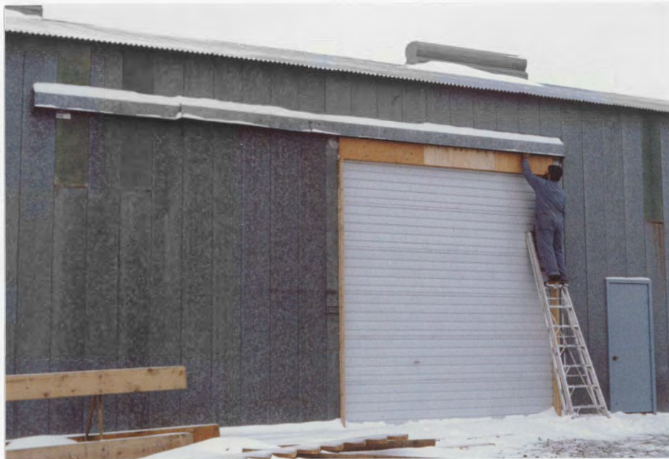
Maintenanceman Humerick finishes the framing in of one of the new warehouse doors.
