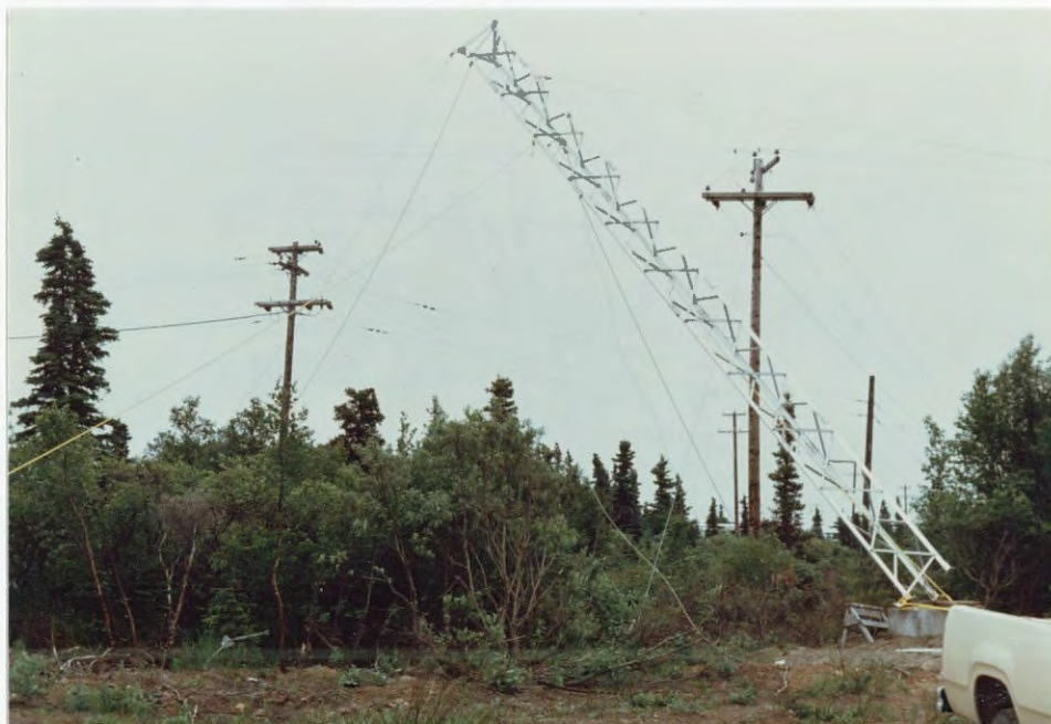
YCC's "erector set" project. Enrollees assembled two 40 foot antenna towers and assisted in their erection.
