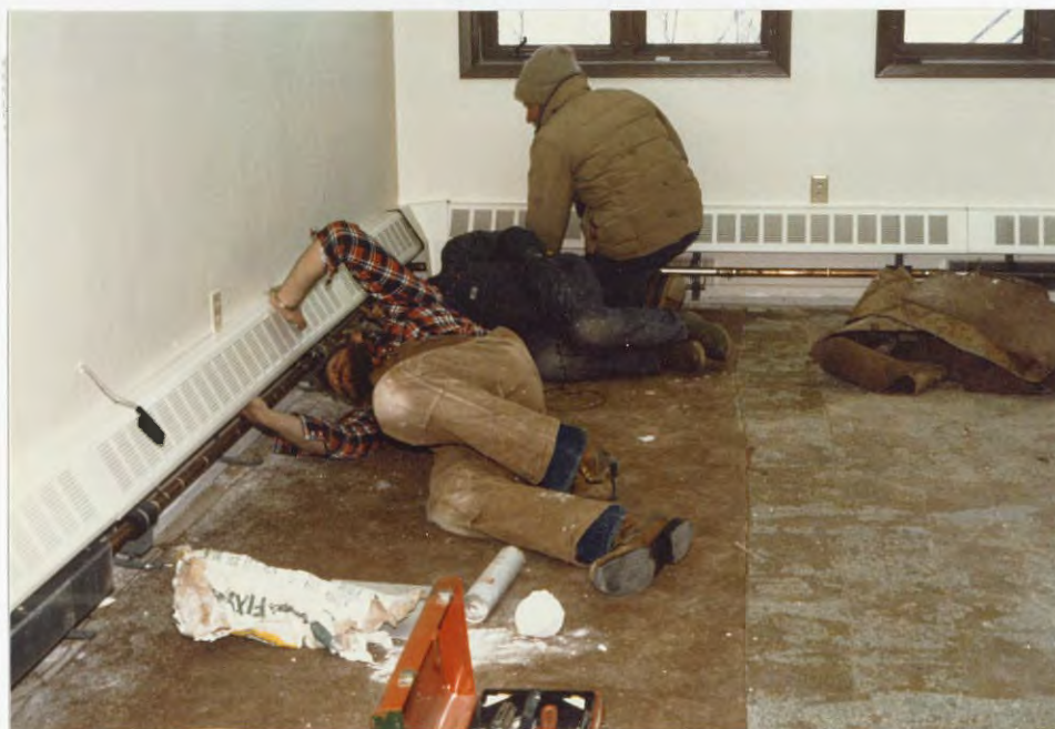
Contractors plumb the radiators in the rehabilitated office/warehouse.
