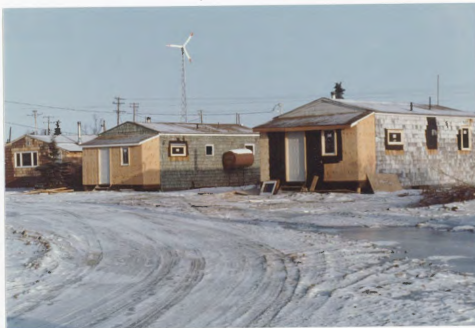
The refuge's 4 kw Enertech wind generator was erected just north of the seasonal cabins under rehab. Standing 60 feet tall in "downtown" King Salmon, the generator is quite a landmark.
