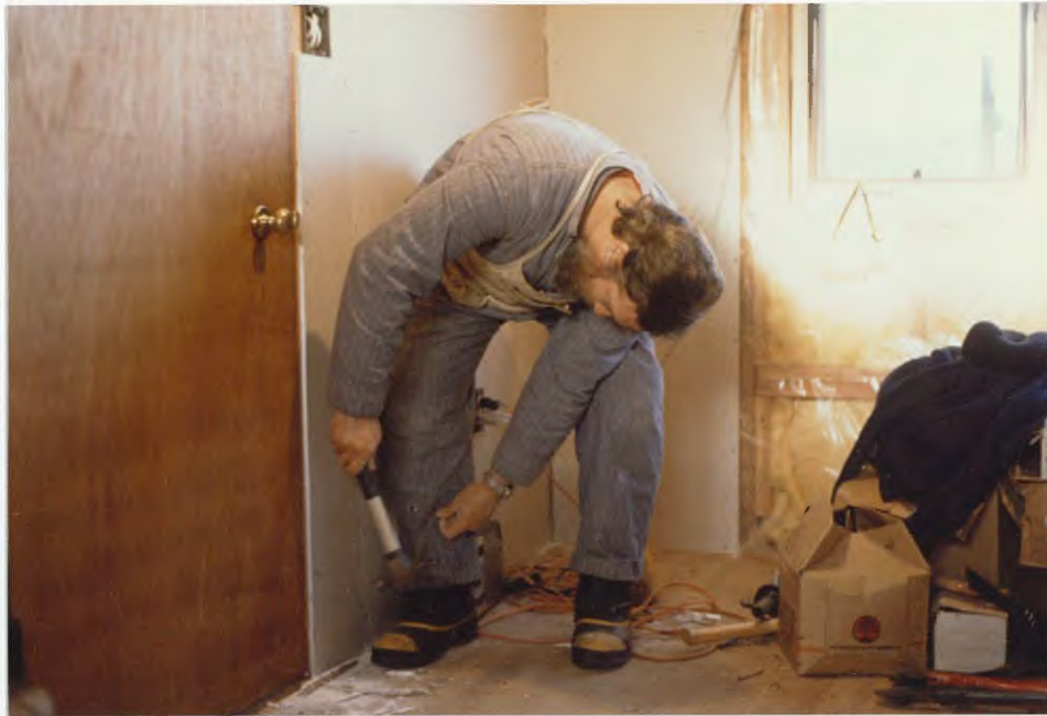
The refuge's two seasonal cabins are in the process of being converted into year around residences. Here Maintenanceman Humerick puts up the sheetrock after insulating.
