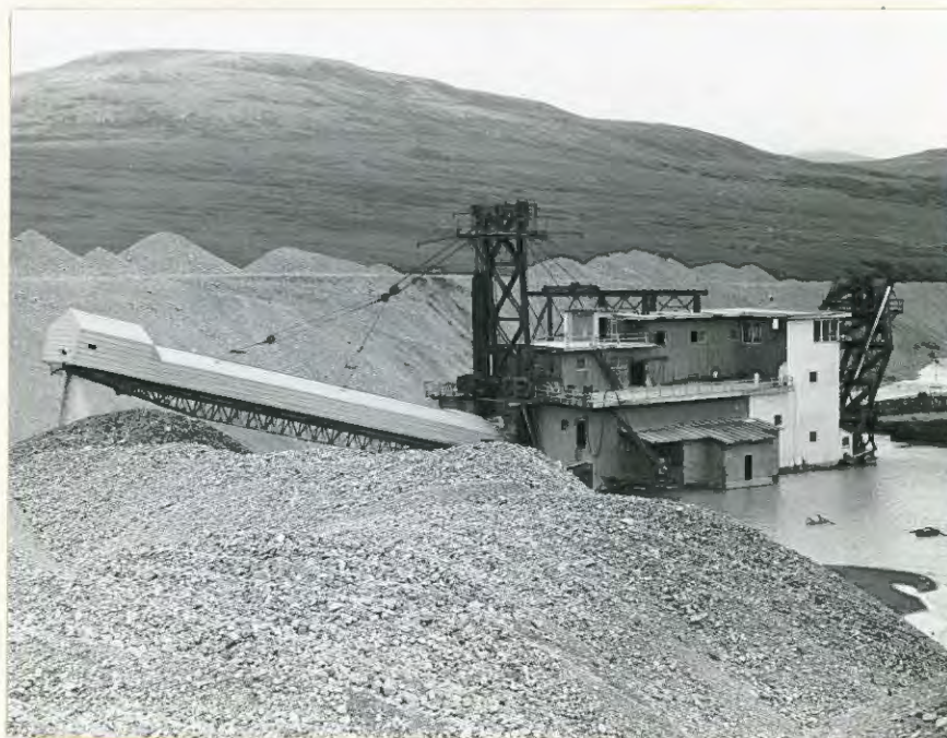
A dredge built at a cost of one million dollars in 1937 is used to extract the platinum and gold ore at bedrock level in the Salmon River.
