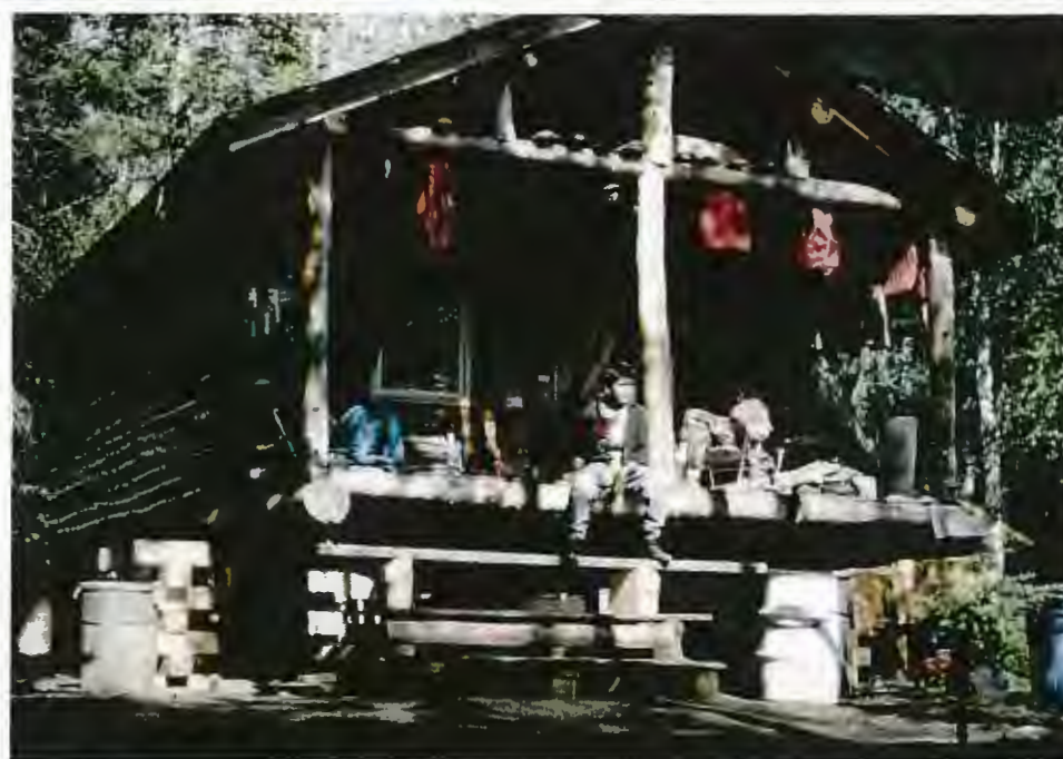
Using cribbing, Small Engine Mechanic Reid raised the cabin over four feet to prevent further flood damage. (KE 8/94).
