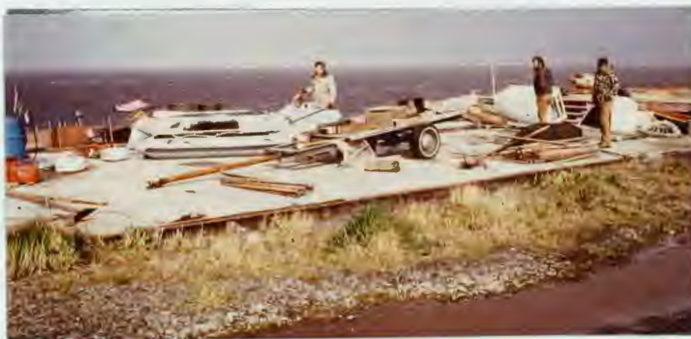
Winds of over 100 MPH lifted the building from its foundation and —
