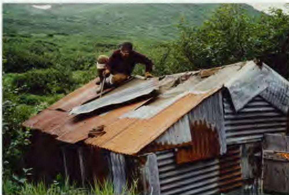
The first step is to remove the sheet metal, as A.R.M. Nunn is doing. (389) 14
