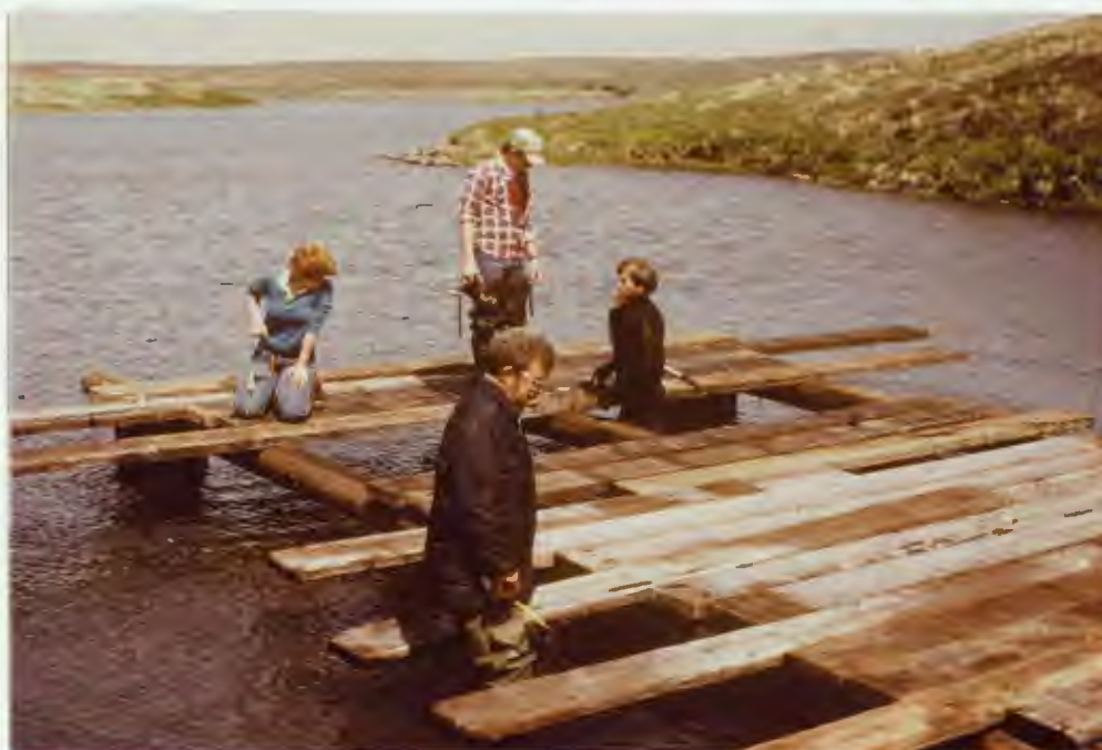
Our float plane ramp at Blinn Lake was constructed of treated lumber salvaged at no cost from the local area. YCC enrollees worked on the project throughout.
