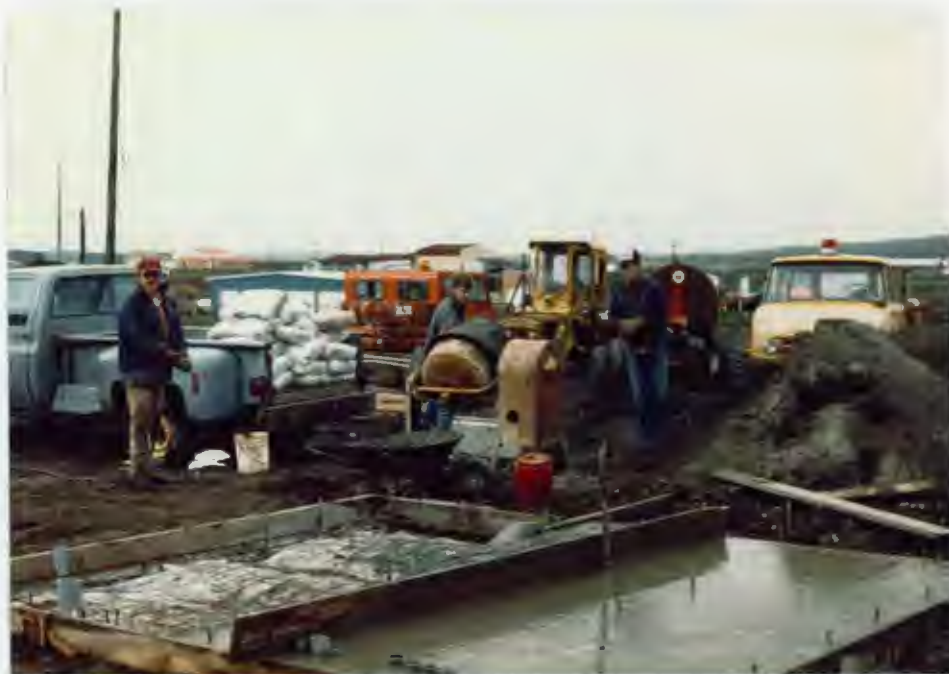
MW Bates and YCC crew laying the foundation of our new electrical switching and emergency generator building. (Blenden)
