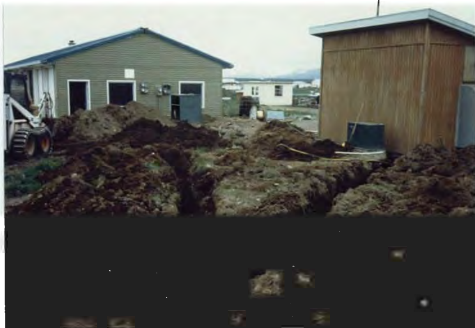
An extensive trenching, wire re-routing job was necessary to put the new headquarters switching facilities on line. This project remedied several substantial safety concerns and ended recurrent problems with outages.
