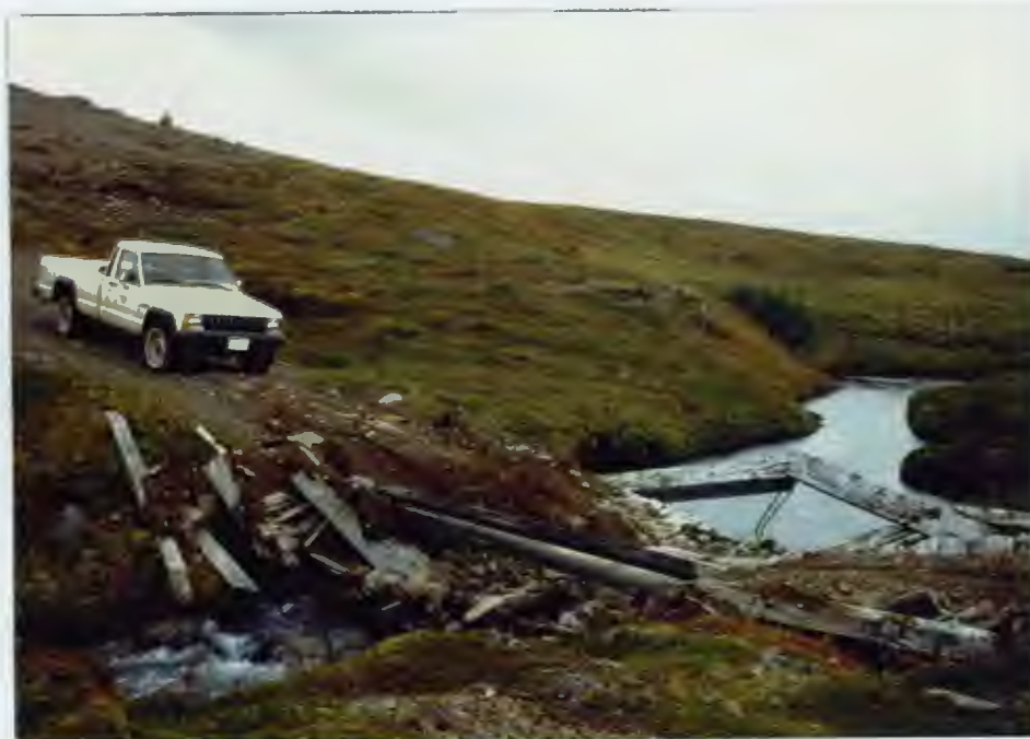
The 4th bridge near the end of Frosty Road, south west of Cold Bay, was collapsed by a local resident driving to heavy a vehicle. Plans are being formulated to either replace this bridge or close the road to vehicular travel at that point.
