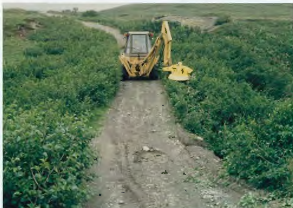
"Brushwhacker" attachment at work widening refuge public use roads 26 July 1993 CFZ
