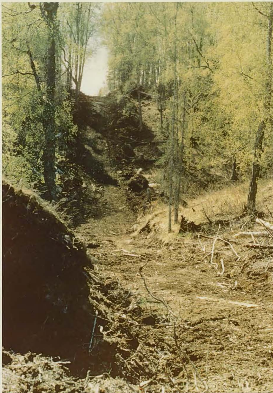
2A-45 Although seismic operators have strict instructions not to disturb sub-surface soils, cuts such as this have occurred.
