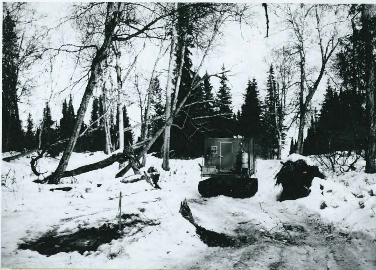
2A-47t Seismic recorder on line just beyond a shot hole. Photo by Richey.
