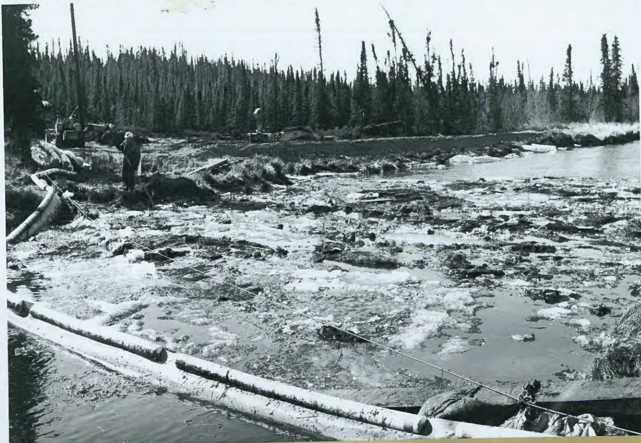
Containing oil spilled from a pipeline break on the bank of the river. Logs on land and across the water prevented pollution from spreading down stream. Workers were coupling on a high pressure line and the oil was being pumped to the sea.
