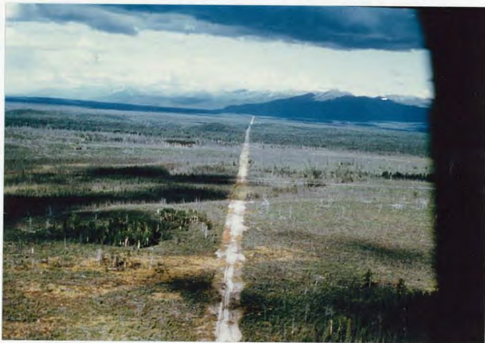
Alaska Pipeline Company 50-foot right-of-way supports two natural gas transmission lines crossing 40 miles of refuge lands to Anchorage Basin users. (Staff Photo)
