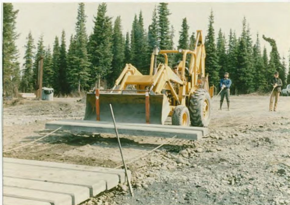
Cement boat ramp, replacing old WWII aircraft landing mats, being maneuvered into place. (7/84, BRC)
