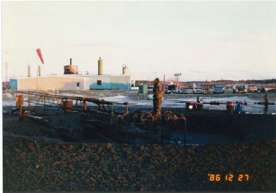
The gas blow out first surfaced from the cellar of well SCU 44-8, depositing subsurface sands, produced water, and some crude around the well pad. RR.
