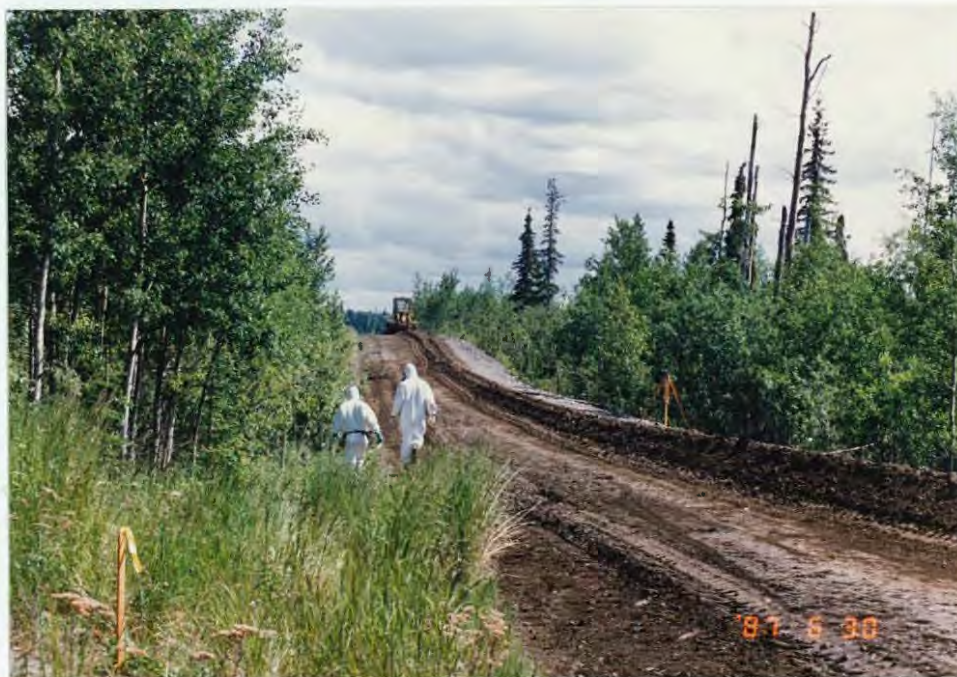
Polychlorinated biphenyl contaminated road gravel was excavated in rows to facilitate recovery operations.
