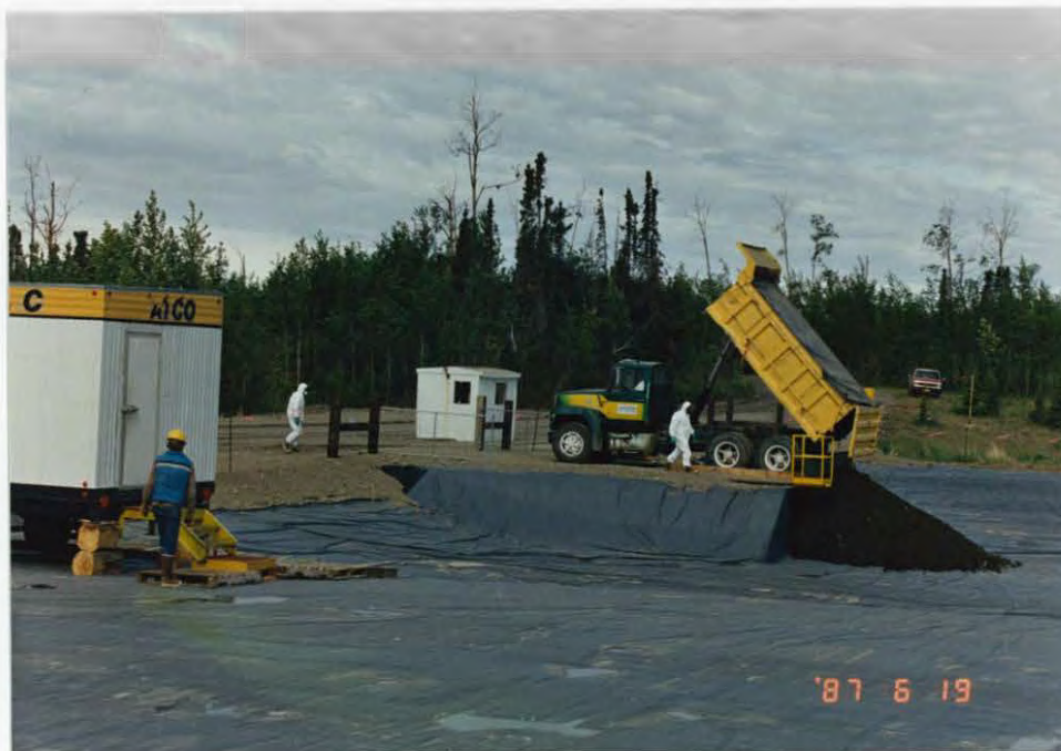
The first load of contaminated material was dumped into the lined stockpile immediately adjacent to the future processing site facility.
