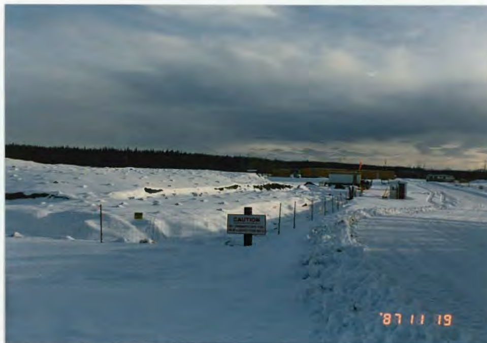
Awaiting processing, the contaminated material stockpile was covered with a Shelter-Rite liner and sandbagged to weather the winter season. RR
