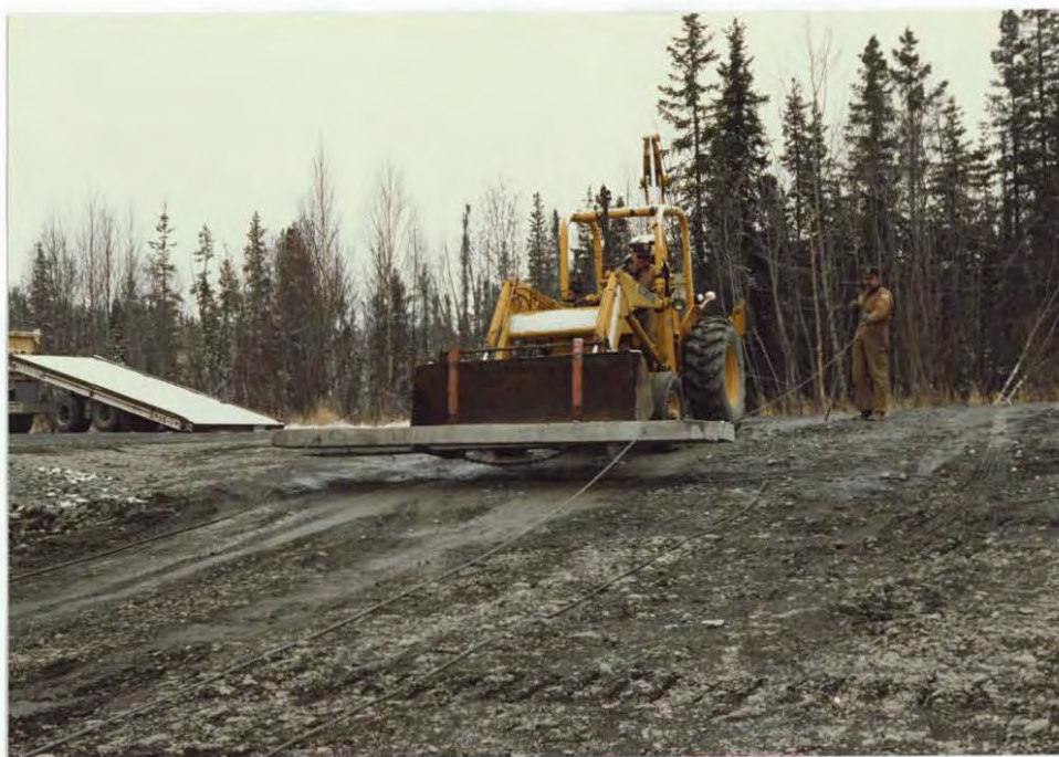
Equipment Operator Kivi and Maintenance Mechanic O'Guinn "stringing" 12' X 12" concrete plank for Lower Skilak boat ramp. JEF
