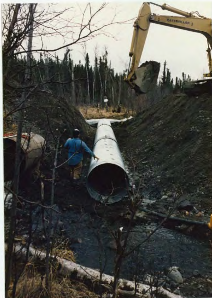
Installation of new 48" culvert on Swan Lake road at Sucker Creek crossing. The new culvert replaced an old "perched" culvert which seriously restricted salmon and rainbow smolt migration into Sucker Lake. JEF
