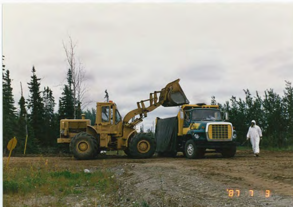
Excavated gravel was trucked to the contaminated material stockpile area for future processing.
