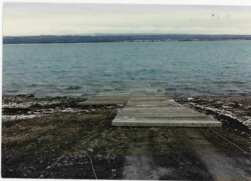
Partially completed concrete boat ramp at Lower Skilak landing.
