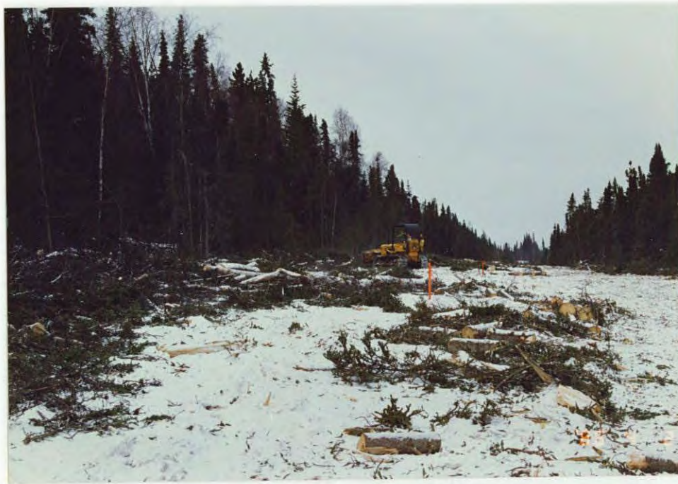
Clearing began March 1986 adjacent the Refuge Headquarters Complex in support of the new Fritz Creek-to-Soldotna 115kV right-of-way.
