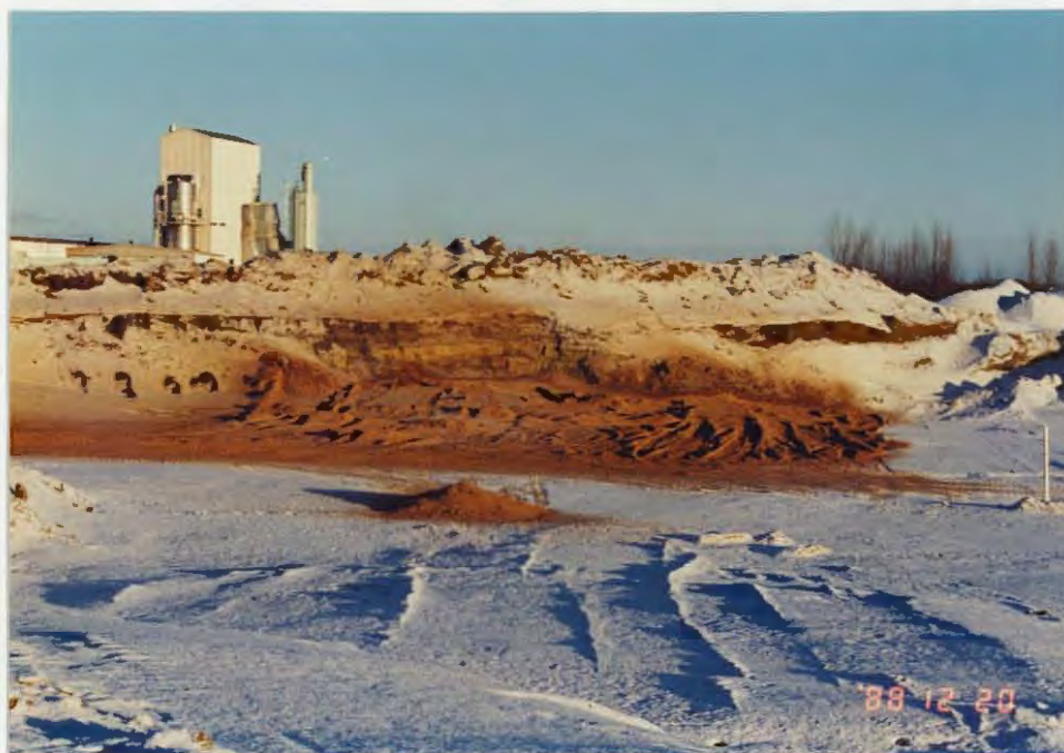
Processed contaminated soils from the Circulating Bed Combustor are disposed in the reclaimed 14-3 holding facility. Note the Combustor's winterized enclosure.
