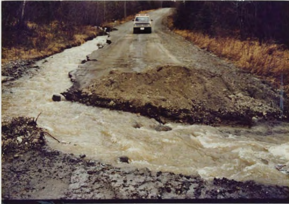
The Upper Skilak Lake Campground access road received extensive damage when the snow-melt caused Lower Ohmer Creek to flood its banks. RKJ
