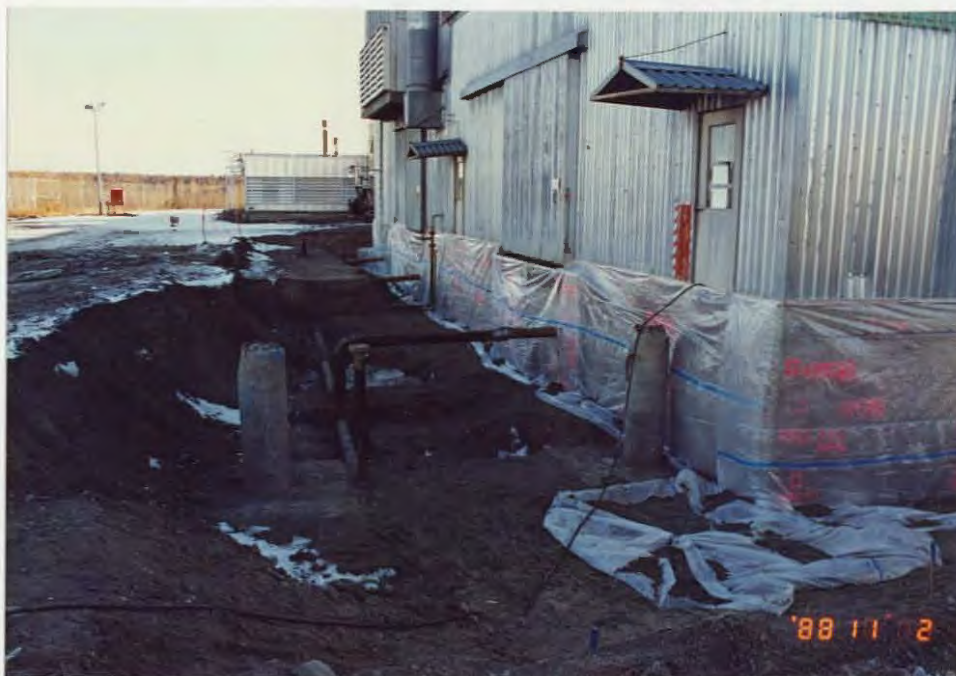
Although contaminated soils adjacent to buildings were removed, numerous wipes of building concrete foundations could not totally remove PCB contamination. RR
