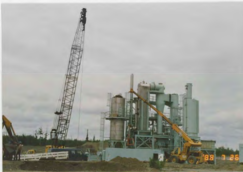
During July, Ogden Environmental Service's Circulating Bed Combustor was erected module by module. RR
