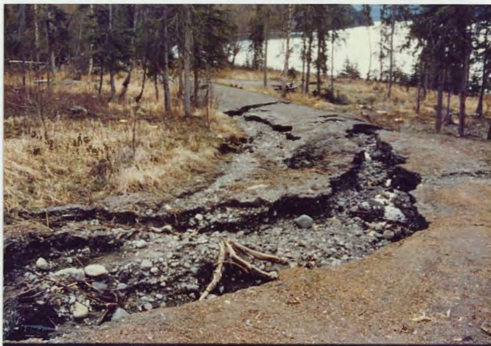
Road and campground pull-outs within the Upper Skilak Campground received significant damage as a result of Lower Ohmer Creek flooding. The new design work for the Upper Skilak Campground would prevent such flood damage in the future. RKJ
