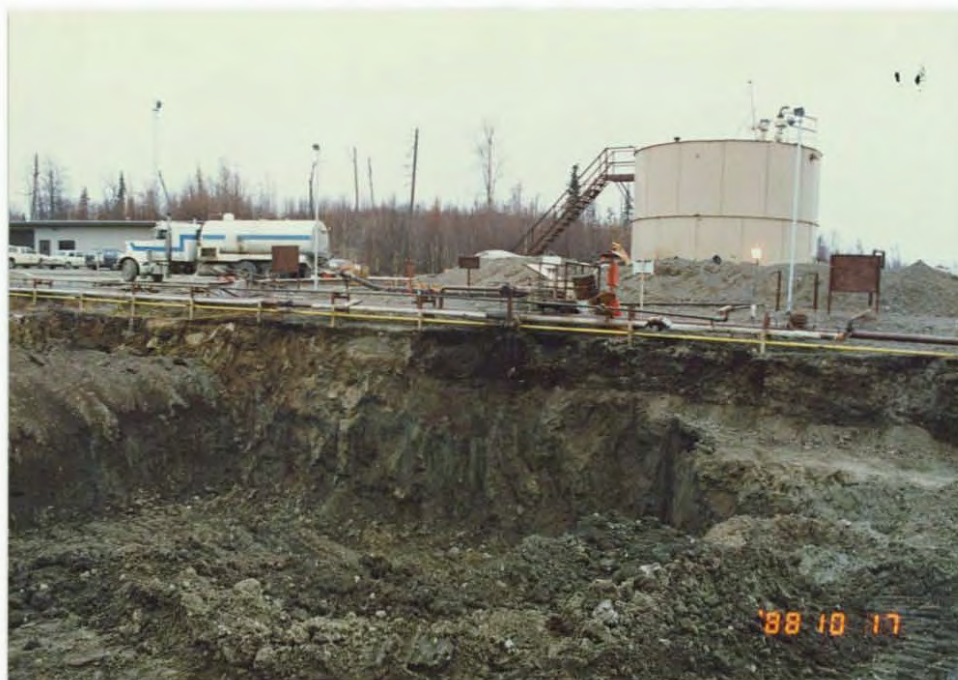
Displacement of crude oil holding tanks and excavation of more than 3200 yards of contaminated soils was accomplished at the Beaver Creek Field prior to winter freeze-up. RR
