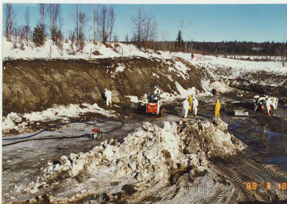
Excavation of contaminated PCB soils began in March, 1988, at the SCU 14-3 waste holding facility. RR
