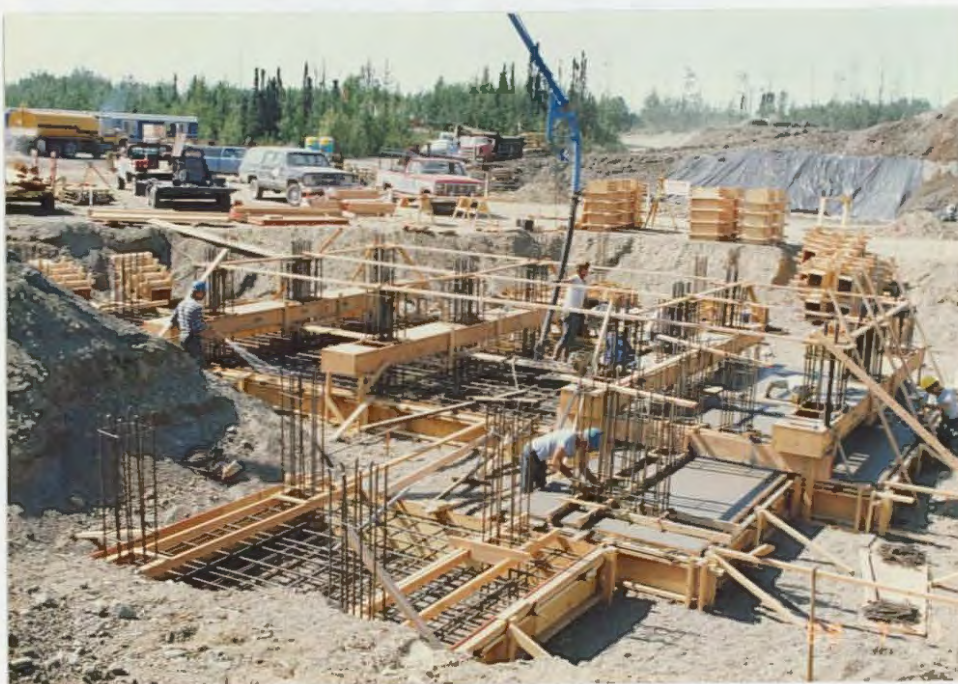
The Circulating Bed Combustor requires a substantial foundation to properly support the facility. RR
