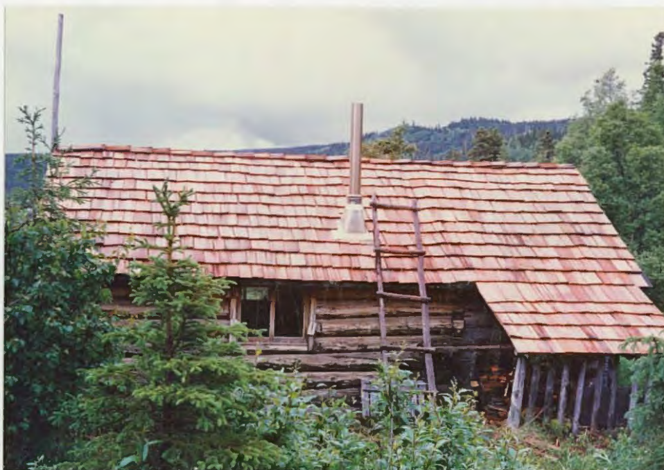
New stovepipe, flashing and cedar shakes were added to the Lake Emma cabin. JEF
