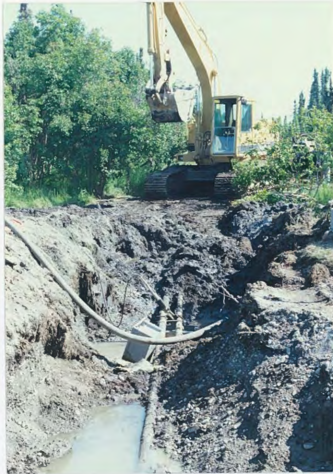
Uncovering old 4-inch crude line across Swanson River. This line was replaced with new 4-inch line with isolation valves located on both sides of river for added protection against leakage. 11/90/JEF
