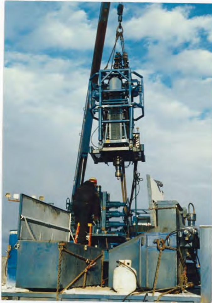
Coil tubing unit being affixed to well head 31A-16 during "plug and abandon" operations at that site. 9/90/JEF
