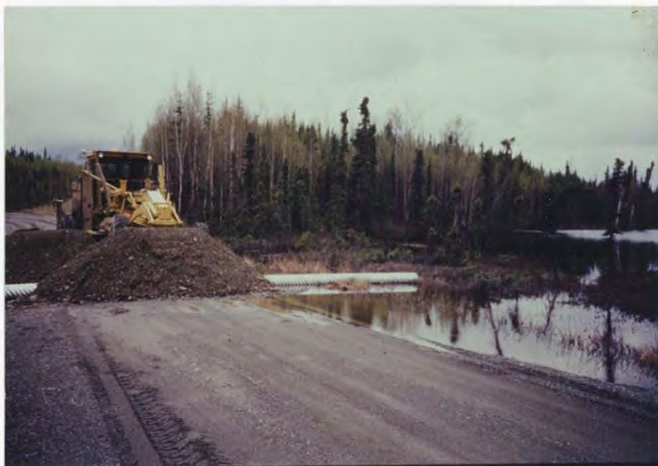
Installation of new culvert on Swan Lake Road near Willow Lake.
