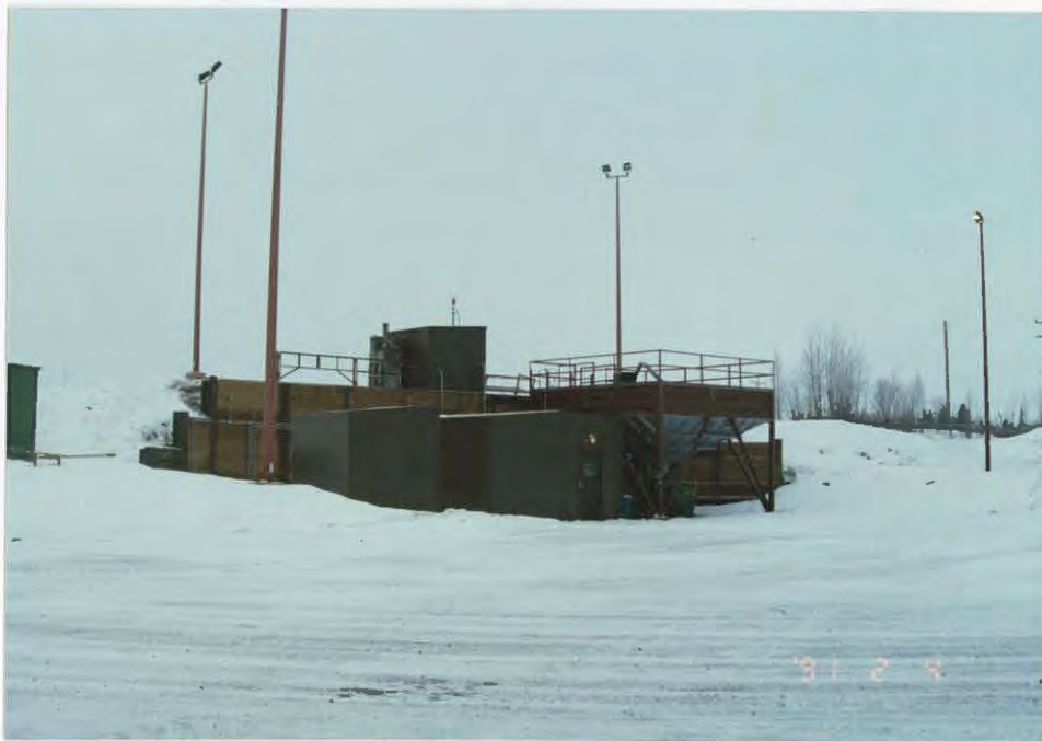
New drum and equipment washing facility near TS-133 at SRF. This "high tech" unit separates impurities from crude, and then pumps it back into production pipeline. Other wastes are trucked to a solid waste disposal site, which became operational in December. 1/91/JEF
