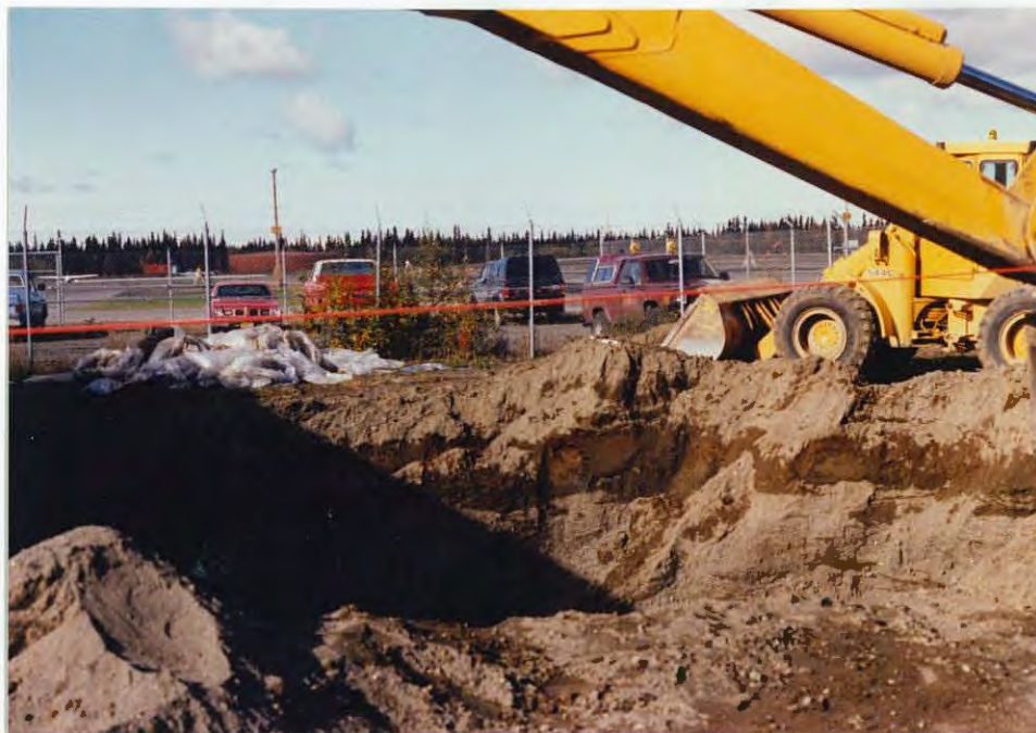
Excavating 2000-gallon fuel tank at old Kenai Refuge Headquarters. No leakage detected! 8/90/JEF
