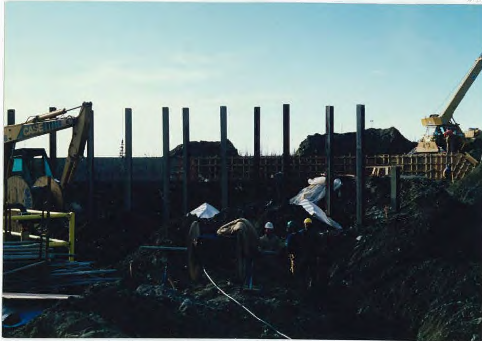
Construction of drum and equipment washing facility at SRF. Replaces old skim or "snake pit" at tank setting T-33. 9/90/JEF
