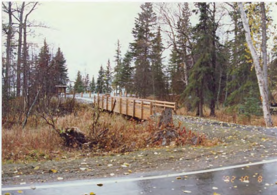
New foot bridge at the Upper Skilak Campground. 92/JF
