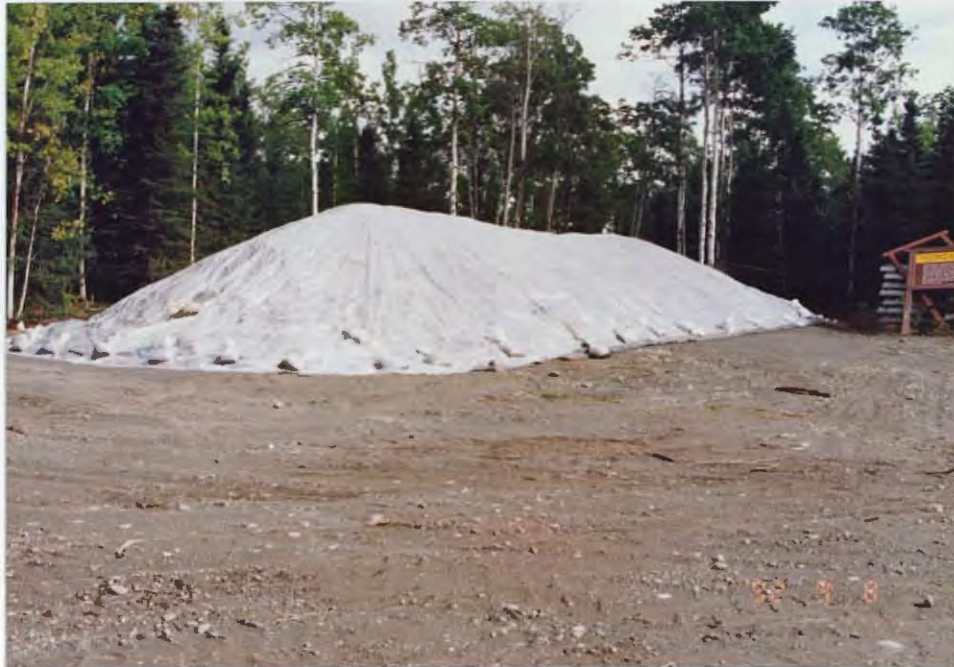
Stockpile of hydrocarbon-contaminated soil at Skilak Guard Station Drum Repository Facility, 1992. Material will be spread and aerated next summer. 92/JF
