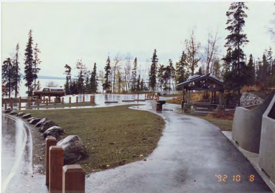
Recently completed Upper Skilak Campground parking area. 92/JF
