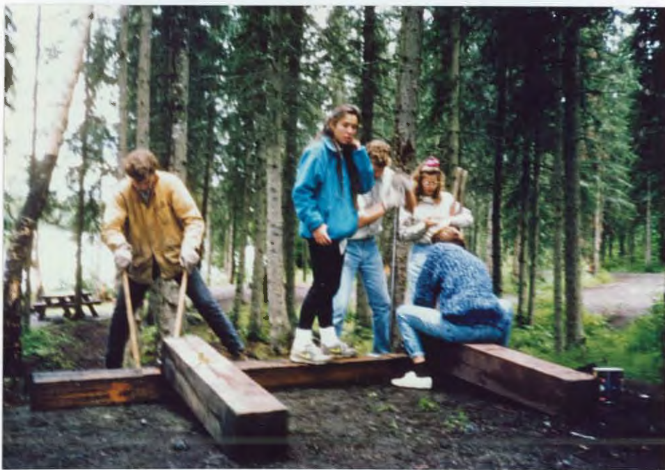
Parking bollards were installed at Dolly Varden campsites. 8/92/SS
