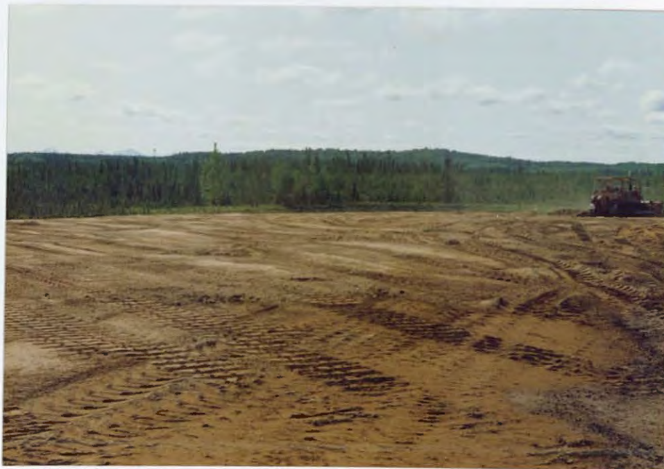
Stockpile of purified soil from the PCB incineration project - a total of nearly 107,000 tons of soil was processed through the incinerator. 92/JF
