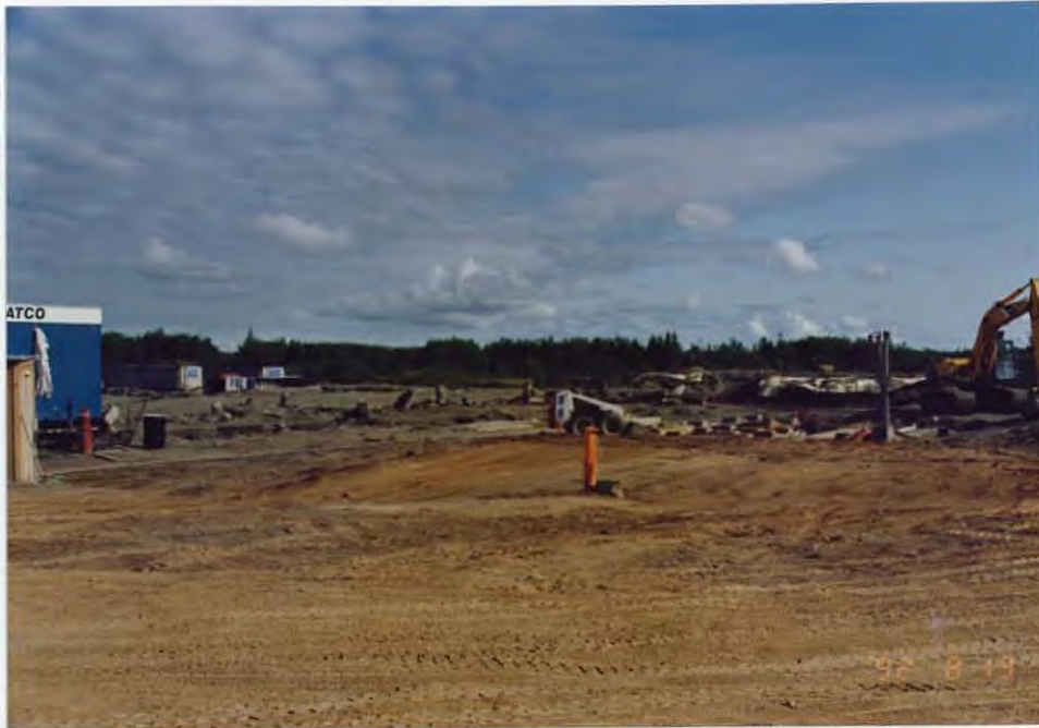
Demobilization of the PCB remediation site at the 14-3 gravel pit. 92/JF
