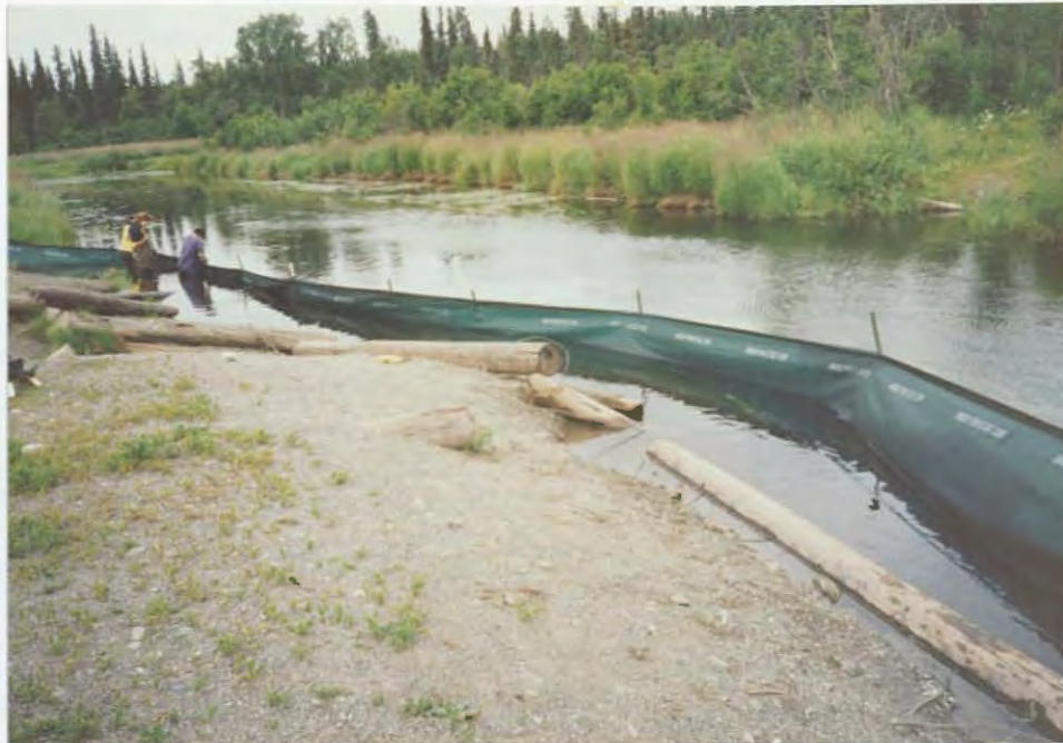
Swanson River Landing terminus prior to renovation project. 92/JF
