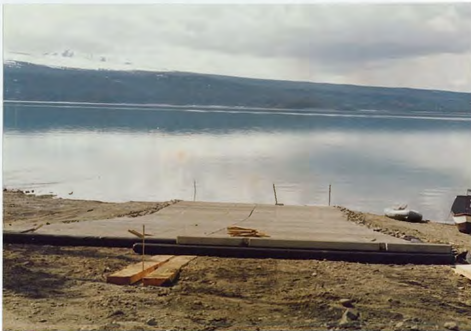
Partially completed boat ramp at Upper Skilak Campground. 92/JF
