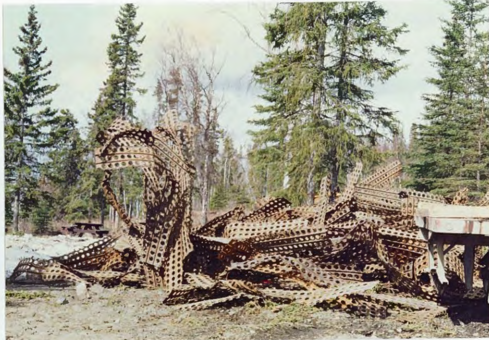
Old military landing mat removed during construction of new Upper Skilak Campground boat ramp. 92/JF
