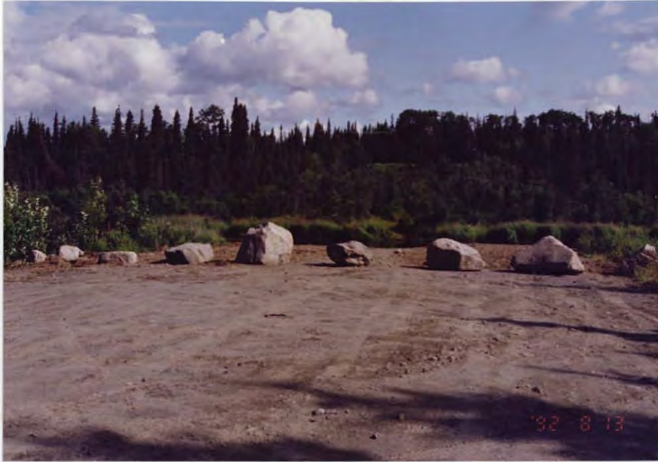
Rock barriers were placed to prevent vehicles from driving to the water's edge at the Swanson River Landing. 92/JF
