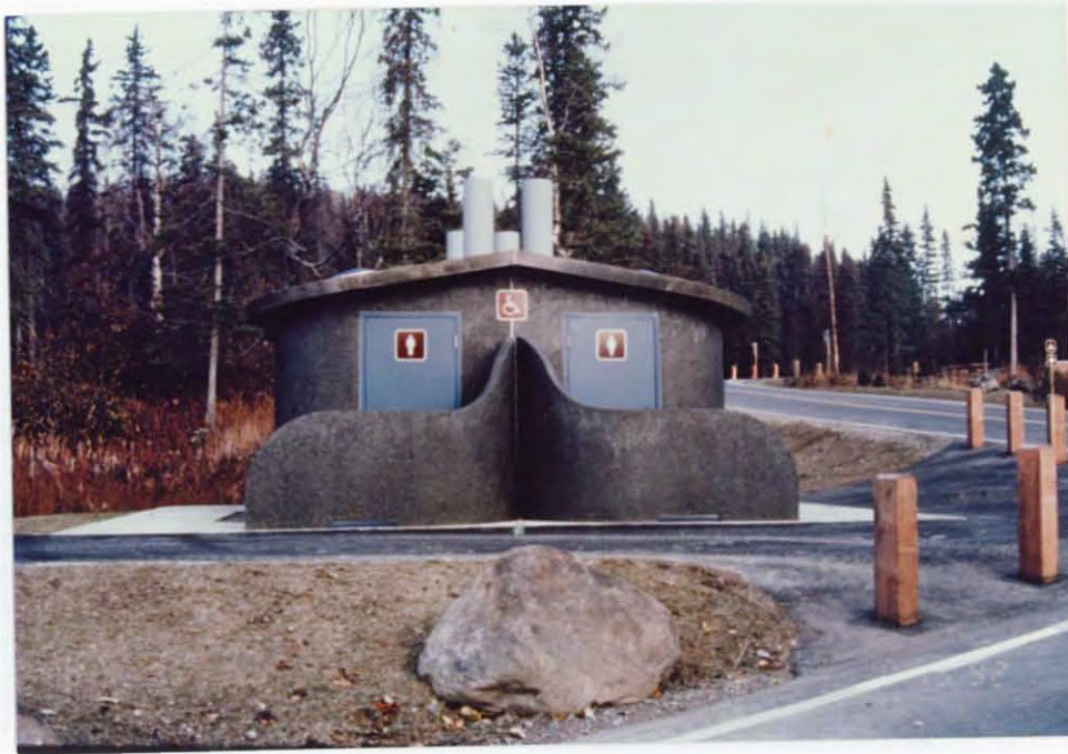
New "concrete bunker" restrooms at the Upper Skilak Campground are expected to be largely maintenance free. 92/JF
