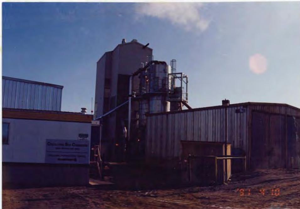
OES's CBC probably holds the world's record for tonnage of incinerated PCB-contaminated soils. 92/JF
