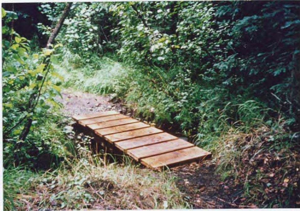
YCC constructed a footbridge on Skilak Lookout Trail. 92/SS
