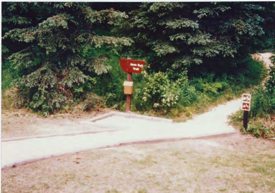
YCC improvements to Keen-Eye Trailhead will assist visitors in the Headquarters area. 6/92 SS
