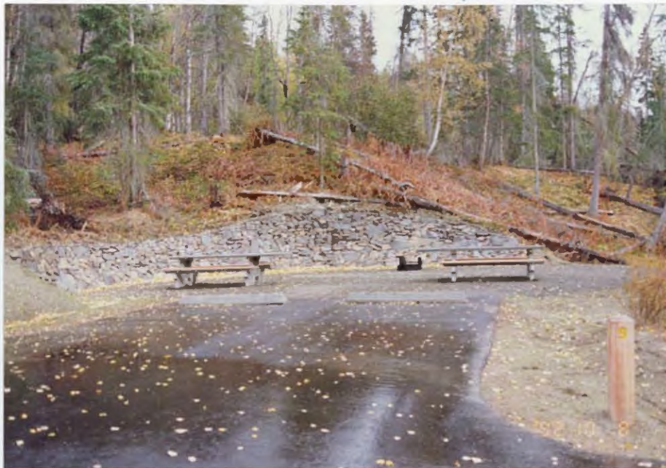
Individual camp sites - Upper Skilak Campground renovation project. 92/JF
