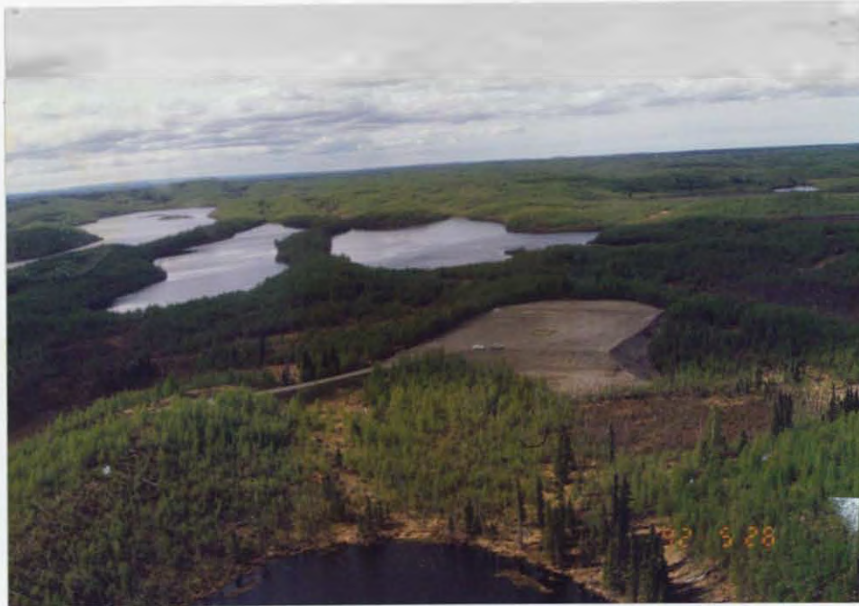
The Galena exploratory well pad in the Finger Lakes Region will be the base of operations for a new exploratory well two miles southwest of the pad. 92/JF
