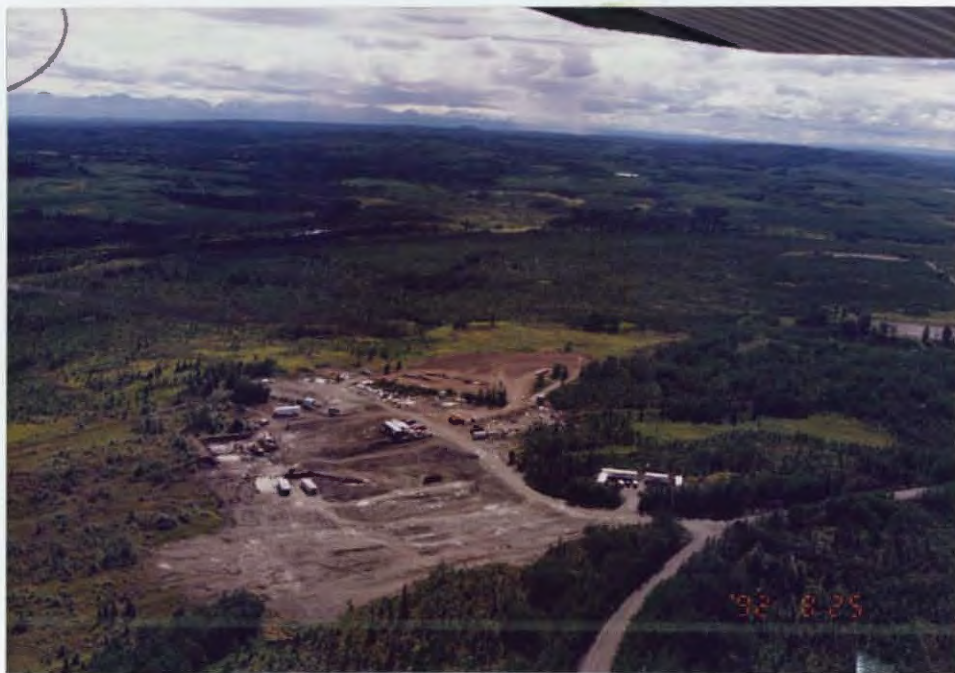
Final stages of demobilization of the PCB incineration project at the 14-3 gravel pit. 92/JF
