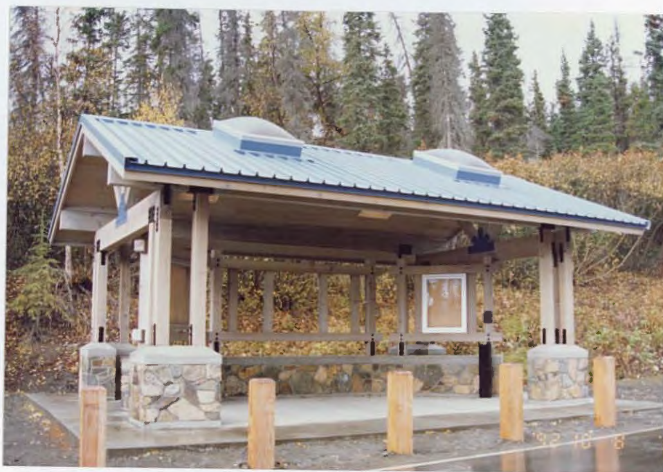
Picnic shelter - Upper Skilak Campground renovation project. 92/JF
