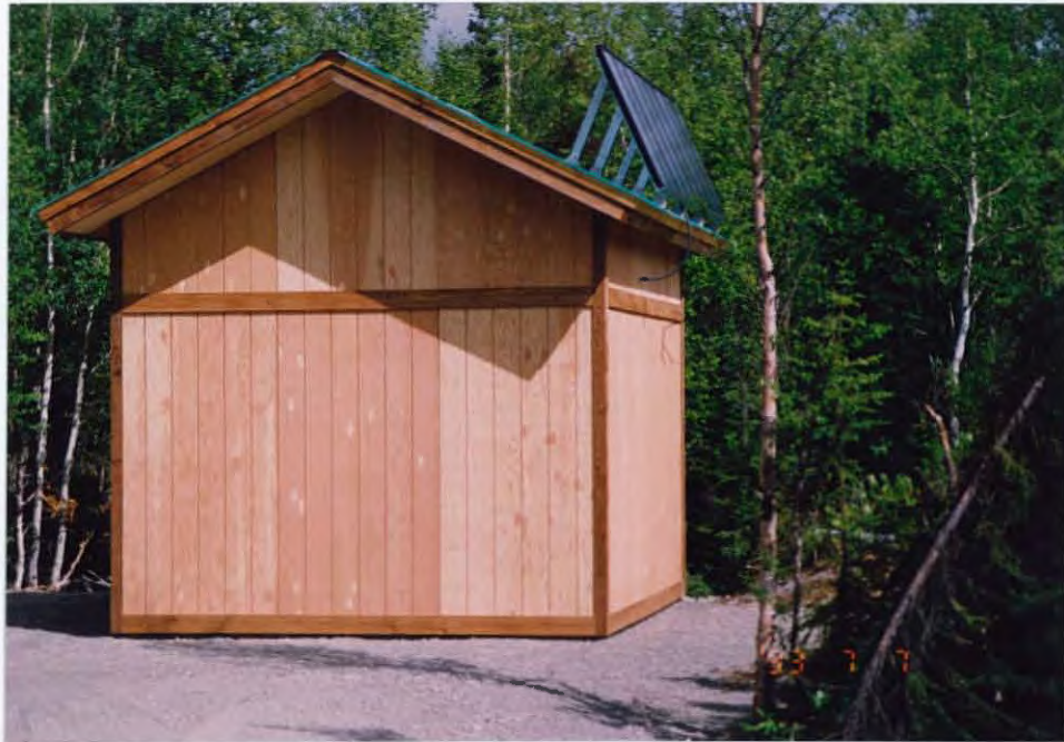
This 12 x 16 foot building houses a solar powered unit for the submersible well and a 2000-gallon storage reservoir for the RV dump site. 93/JF
