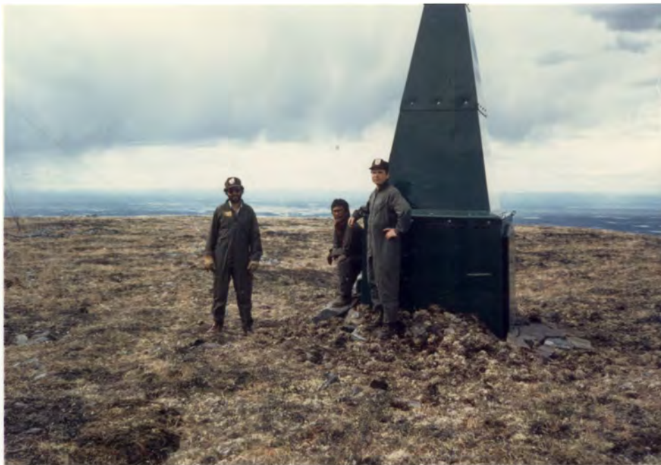
ROS/P Spindler, BT Wholecheese and FMO Granger prepare the site and assembled the new radio shelter on Totson Mtn, 25 mi SW of Galena. New solar panels, batteries and antennas were connected to the old radio equipment. All but the solar panels are contained within the new shelter. Despite these efforts the low bid battery connectors cracked in the cold and radios failed in the fall of 1991.
