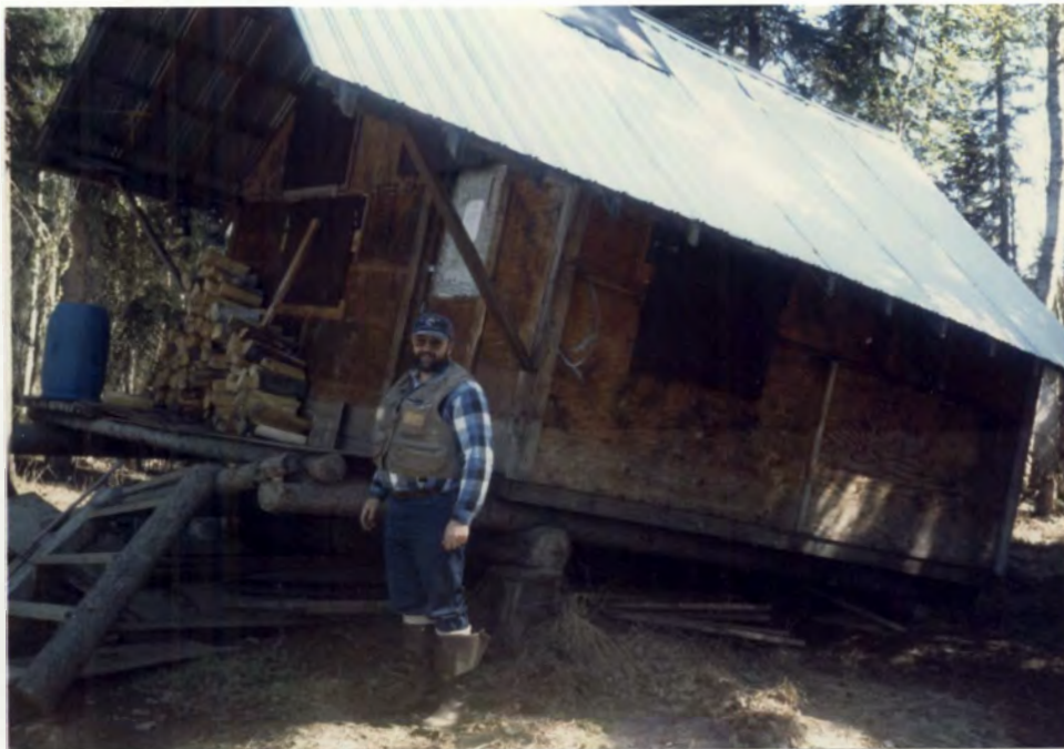
Airplane Pilot Colin "Brownie" Brown and the flood damaged lower Nowitna administrative cabin. An ice jam on the Nowitna River caused flooding on high banks which rarely flood. The cabin was jacked up and leveled back onto its foundation. This cabin was given a major cleaning and painting after the flood in 1991.
