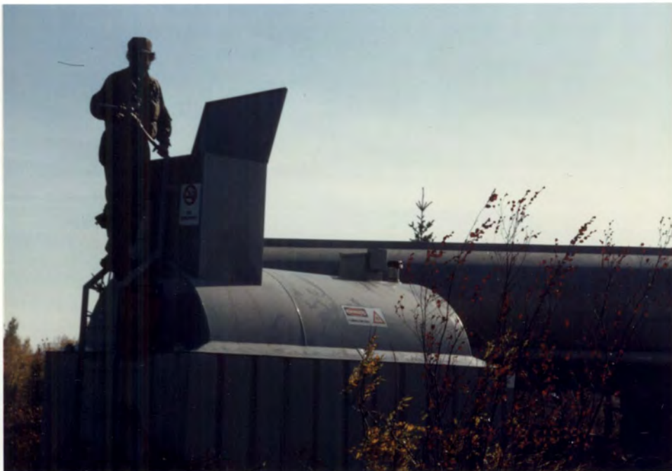
Two double wall 1500 gallon bulk avgas tanks were installed, one at Ruby and one at Huslia. The purposes of the bulk tanks were to make refueling safer and to eliminate as many fuel caches as possible in remote field areas. The bulk tanks are filled once per year by barges originating at the railhead in Nenena.
