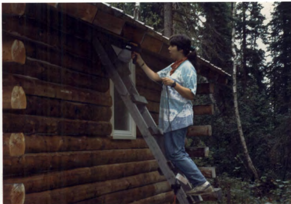
BT Jenny Lowe adds a coat of log sealer to the Hog River administrative cabin. BT's Lowe, Huntington and Wholecheese, along with FMO Granger spent a total of 2 weeks doing maintenance work on the cabin and building an adjacent equipment storage shed.
