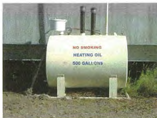
New 500 gallon double-walled heating fuel tanks were installed at each of Galena's six FWS residences. (GM)
