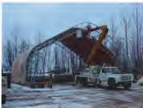
Richard Hannah, Alaska Structures, in City of Galena truck placing rope to pull last sheet of fabric. P Huhndorf to the left holding end of rope. 10/03
