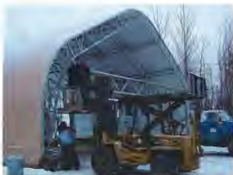
Richard Hannah, Alaska Structures, and WB/P Scotton bolting main overhead brace on west end of airplane storage building. P Huhndorf and MW Strassburg placing post. 10/03
