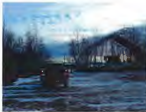
Looking at front (west) end of airplane storage building with all arches in place and one sheet of fabric installed 10/03
