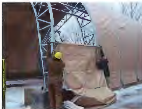
P.Huhndorf and WB/P Scotton getting sheet of fabric started in slots in preparation for pullin over the arches. 10/03
