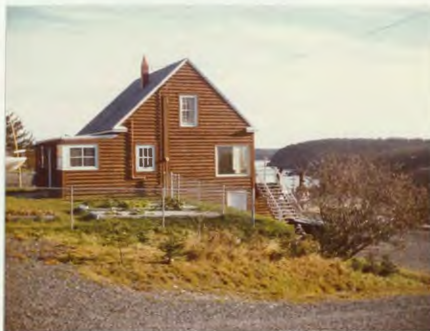
Quarters # 1 after new siding was installed and stained. New chain link fence was installed and grounds cleaned up. A new roof and oil-fired baseboard heaters were installed after photo taken. R.D.
