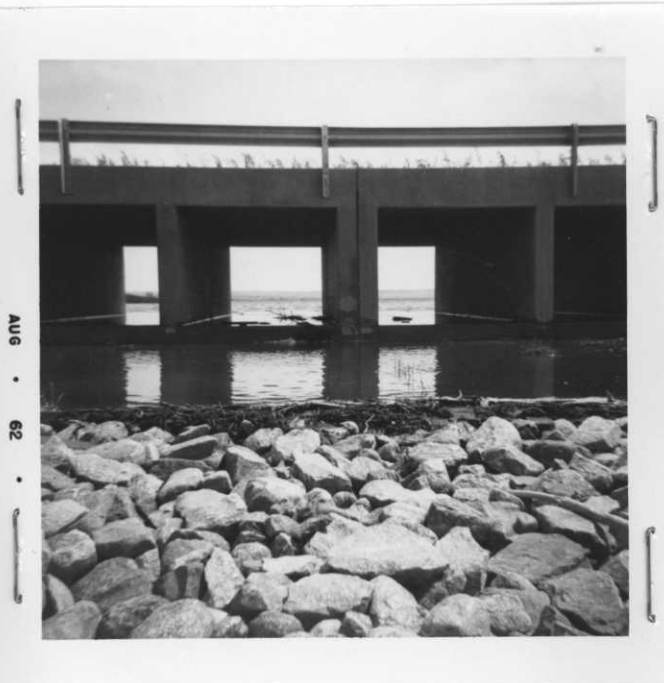
R1 Looking through the spillway in to the refuge. Spillway elevation 1607' - Corps purchased to 1620'. Culverts are 6'X6'.
