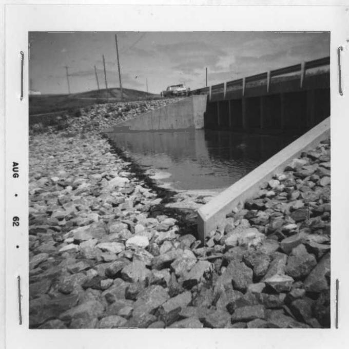
R1 A close-up of the spillway showing the concrete apron and rock rip-rap along the downstream face of dam.
