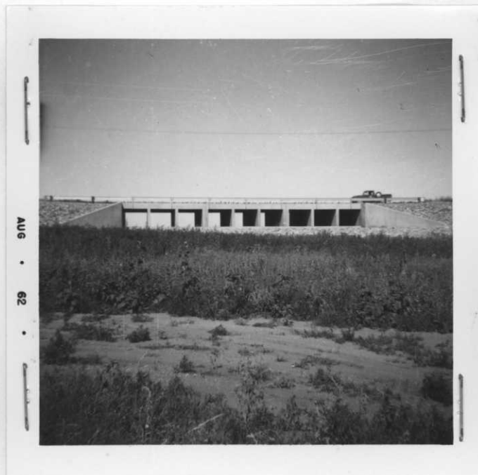
R1 A view of the 9 culvert emergency spillway from the Oake Reservoir side.
