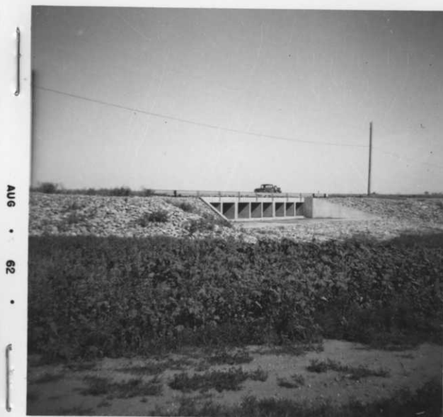
R1 The spillway is designed to take water both ways. This is the Oahe Reservoir side. Rip-rap will protect the dam from washing.
