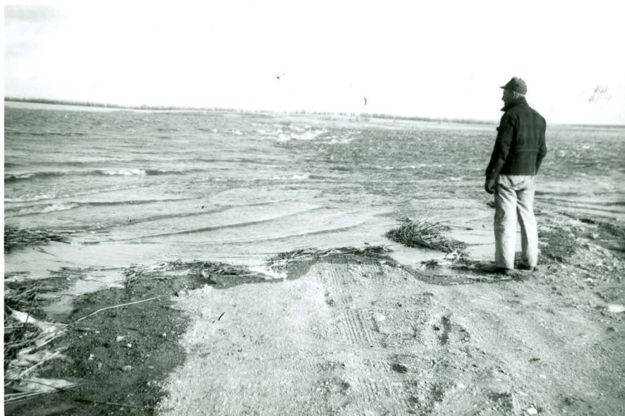
No. 18: Apr. 22 - Water begins to flow freely over the newly constructed emergency spillway at Columbia dam. A head of only 2 to 3 inches prevented serious erosion. E. Kaastad checking.
