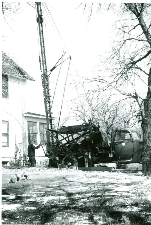
No. 14: March 5 - Surface well drilled at Site 2 to replace failing artesian well. A third well was drilled at our Recreation Area. E. Podoll and E. Kaastad operating.
