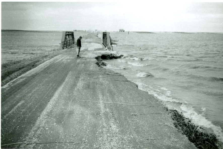
No. 26: Apr. 30 - More flood destruction. High water and waves combine to destroy the Weismantle Grade. E. Kaastad watching. Grade later cut through in many places.
