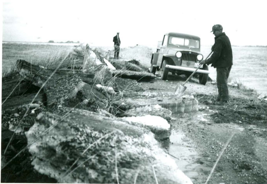
SD-SOL-472 No. 15: Apr. 17 - Spring break-up. Ice 14" thick forced over Mud Lake dike by high wind did considerable damage to the dike. E. Podoll and E. Kaastad.
