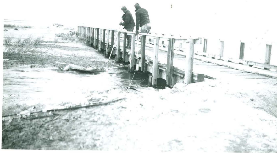
SD-SOL-473 No. 16: Apr. 18 - E. Kaastad and E. Podoll breaking ice jam at Mud Lake bridge to prevent loss of the structure.
