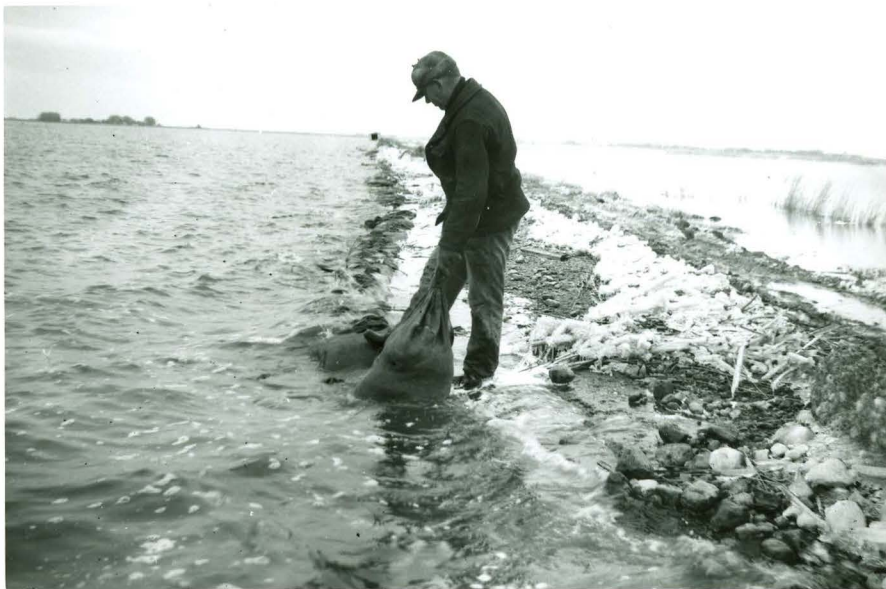
50-50L-480 No. 23: Apr. 27 - Water still rising. E. Podell placing sandbag on Mud Lake dike to prevent channelling. Note the ice which added to our difficulties.
