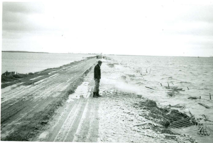
No. 25: Apr. 30 - Flood destruction. E. Kaastad watching wave action take tons of fill out of State Highway #10 (Houghton Grade) where it crosses Sand Lake Refuge. Road badly damaged and closed later.
