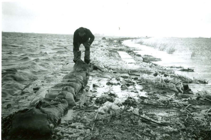
50-50L-481 No. 24: Apr. 28 - Over the top. E. Kaastad placing sand bags to stop channelling as flood water tops Mud Lake dike. Note ice which denotes unseasonably cold weather.
