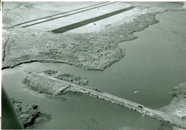
Dakota Lake dam and spillway. Picture was taken from the airplane during waterfowl census. Because this country is so flat, (the James River drops 1 inch per mile) frequent high winds cause flooding, especially when the impoundment is at spillway level.
