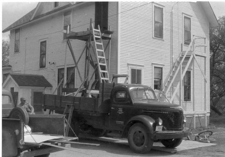
Elmer Podoll's portable scaffold being used to close in the bathroom window of the Assistant Manager's quarters. The maintenanceman lives downstairs.
