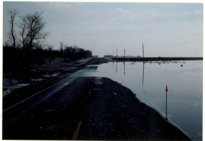
Figure 2. . . . with water "piling up" behind roads with culverts too small to handle the volume of water (Highway 16, south of headquarters),...
