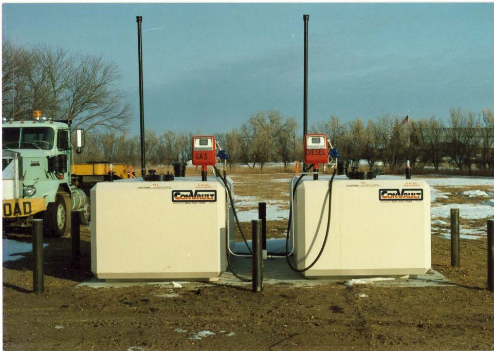
Figure 58. . . . were replaced with two above ground self-containing storage tanks. 89-MJH
