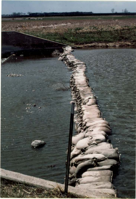
Figure 59. Bureau's solution in capturing additional flows at Dakota Lake NWR, is the use of sandbags for capture and diversion of streamflows to its West Oakes Area Irrigation Test Facility. 89-JWK
