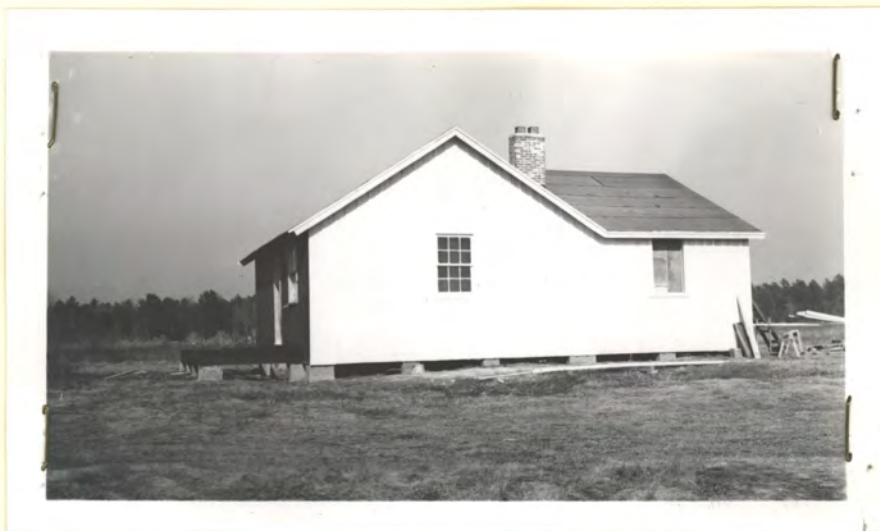
Progress made on construction of dwelling for Tenant Farmer. Floors and sides of house are all double thick with a layer of 15# asphalt felt between.
