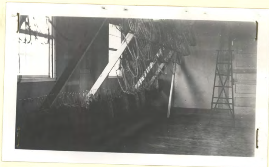
A section of the drying room in the fur house, showing muskrat skins being stretched on lower tiers. Upper tiers contain empty stretchers. Note that muskrat hides are stretched with fur side inside, and are kept parallel so that the flesh sides do not touch, as this causes softness and rot. Taken January, 1941. Exposure 5, Roll 17.
