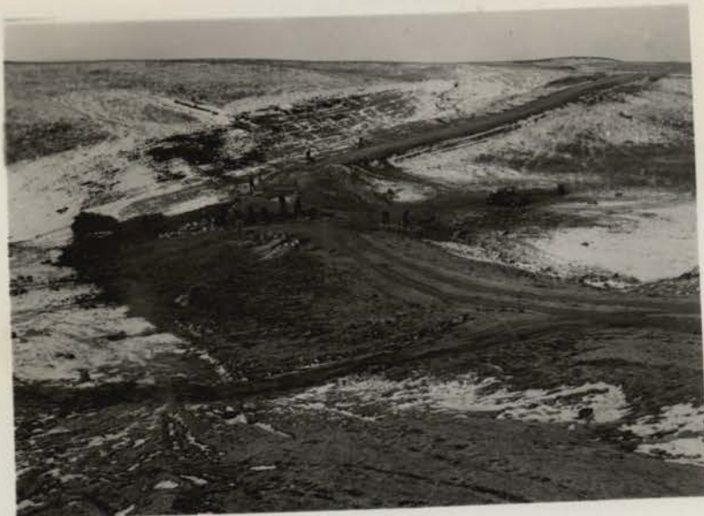
Riprapped fill across the lake from the Secondary Headquarters with a close-up view of the paving of the spillway.
