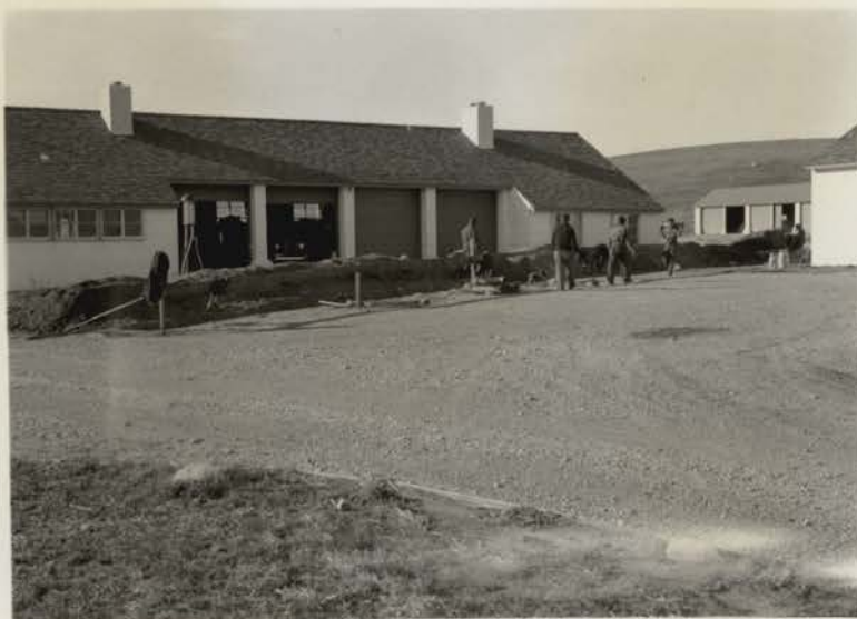
Shingling the roof of the building for which the sewer line has been excavated.
