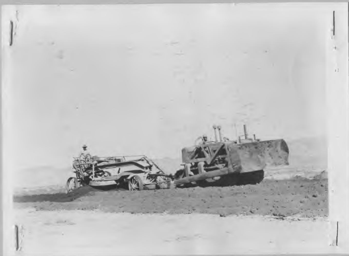
HD-14 and blade breaking down dragline spoil bank for Hunter Road
