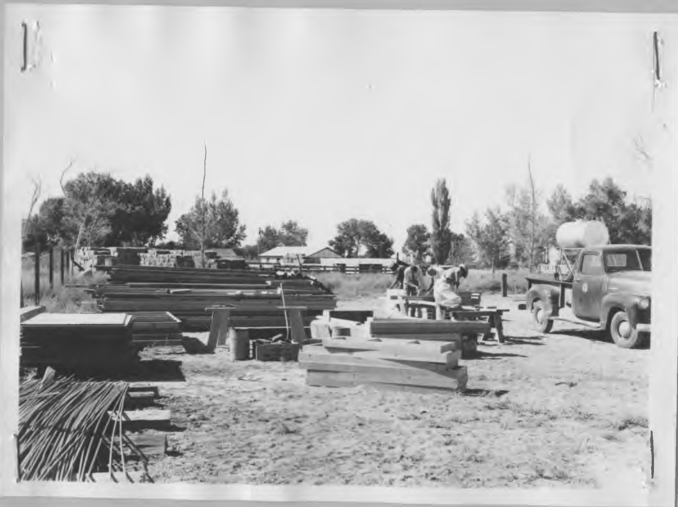
The Concrete Crew assembling forms
