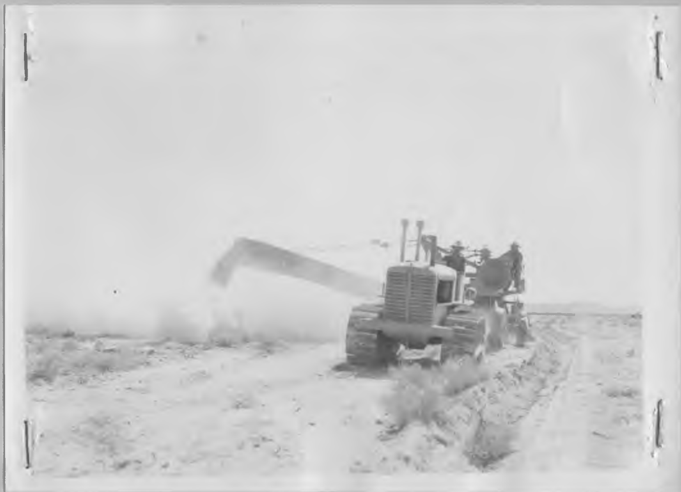
Elevating Grader cut on Palute Canal.
