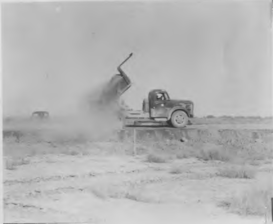
Spreading gravel on Hunter Road
