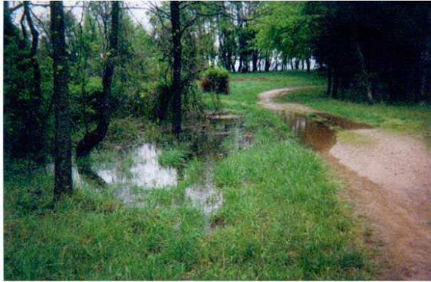
Flooded area before culverts and vernal pool
