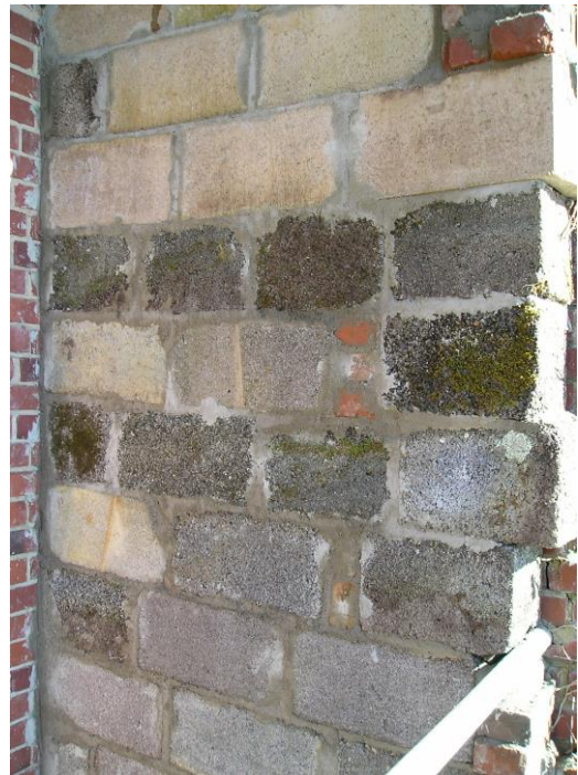
Entrance to Shelter after being sealed
