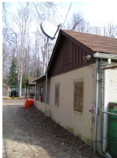
Satellite next to Refuge Shop
