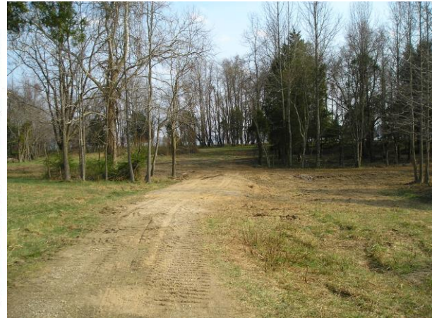
Flooded area after culverts
