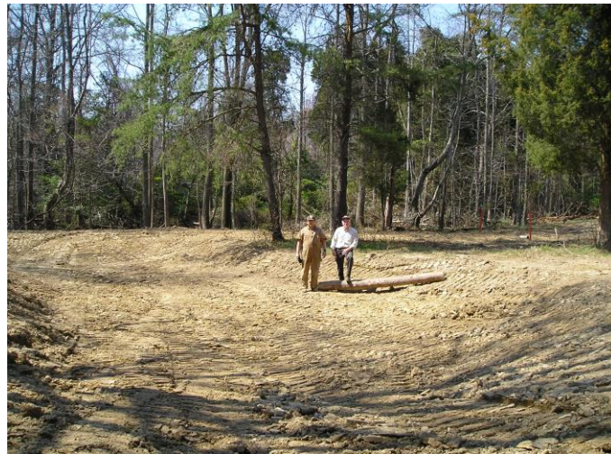
Vernal Pool created for Run-off ( Boska and Witt above standing in vernal pool)
