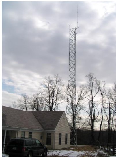
Tower on BLM property
