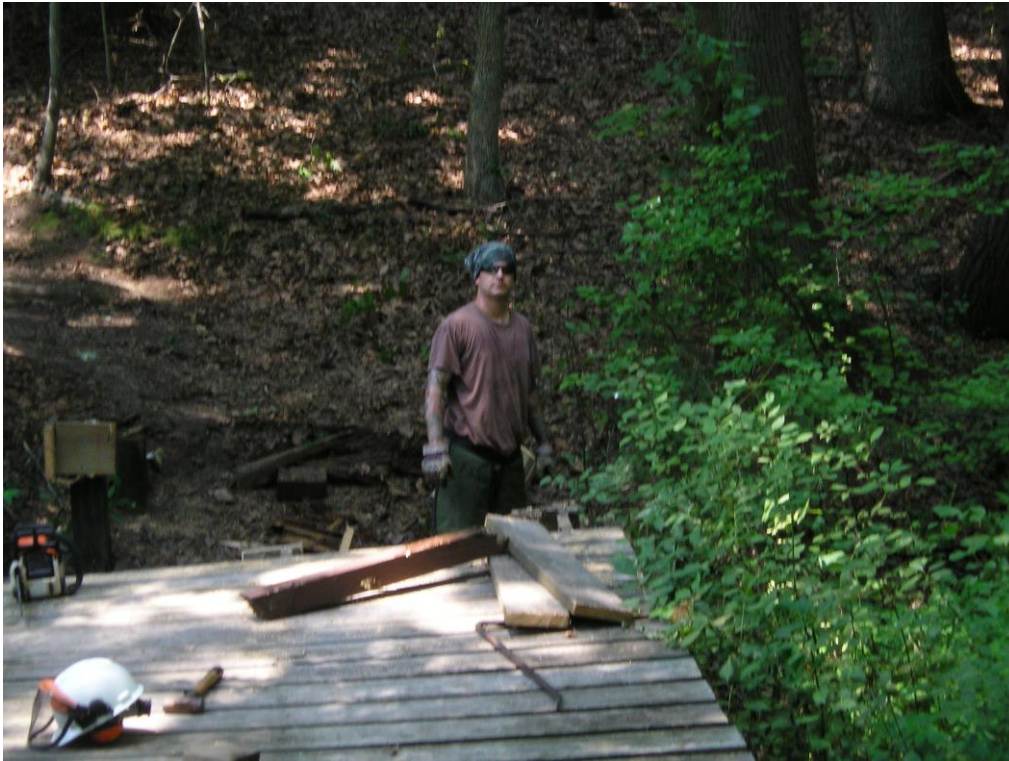
Maintenance Worker Revis removing sections of bridge
