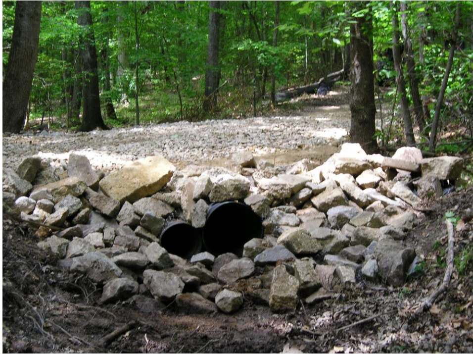
New culverts on Tree Stand Road
