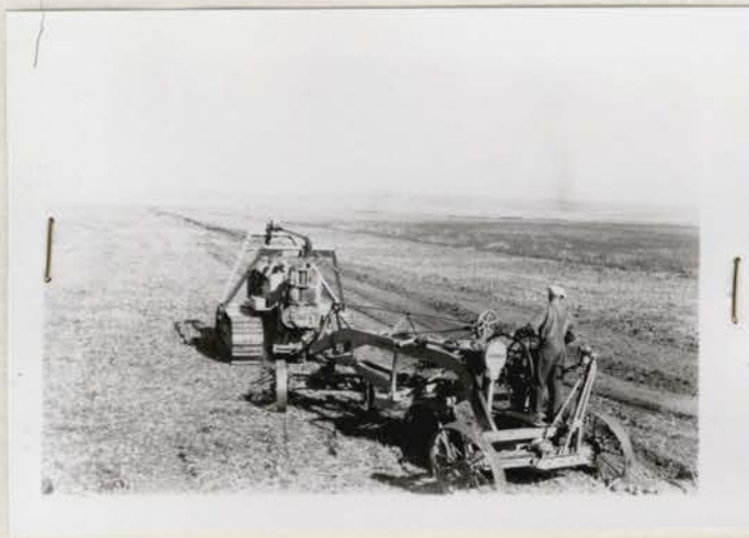
Picture No. 491. Stripping and scarifying ground in preparation for base of dike. August 1940.
