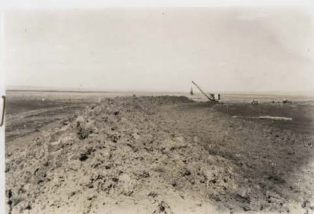
Picture No. 490. Dragline in operation casting dirt for Dike on curve around north side of Great Northern Reservoir near section line between Sec. 31 and 32. August 1940.
