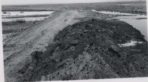
No. 659 Dike fill of about 3,000 yards sufficiently completed to provide for access and transportation of equipment to west side of lake channel. August, 1941
