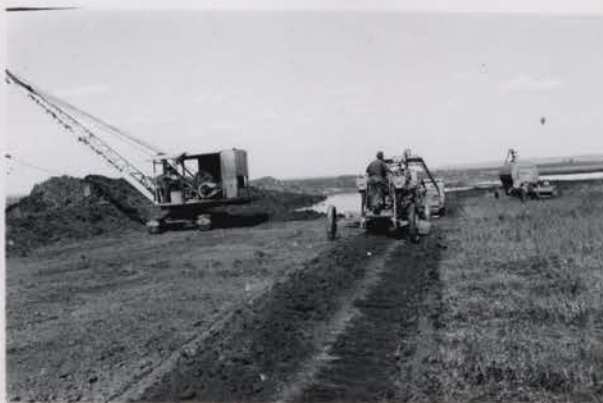
No. 661 Both dragline and Caterpillar, and blade outfit at work west of lake channel on Dike "C". September, 1941
