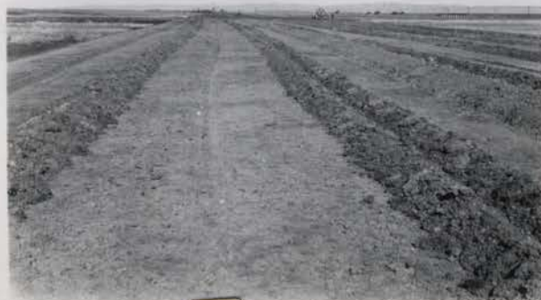
No. 662 Prepared base for Dike "C" south of main Bowdoin lake. Note that all vegetation has been removed and ground trenched to prevent seepage. Dragline, Caterpillar outfit, and town of Bowdoin can be seen in distance. September, 1941
