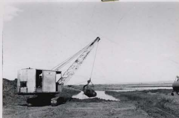
No. 660 Dragline equipment has crossed dike fill across lake channel and is getting under way with continuation of dike "C" to the west. August, 1941
