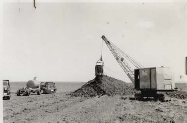
#564 Casting fill for Dry Lake dike.
