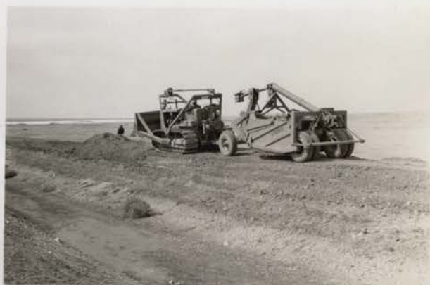
#560 Leveling of dry lake supply canal bank in construction of patrol trail.
