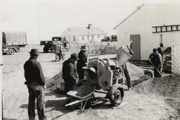
#562 Mixing concrete for equipment building floors.
