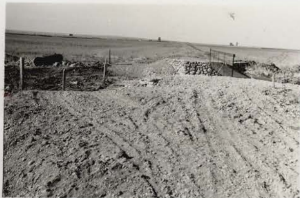
#556 Cat-walk and graveling top of wing-wall fills completed on 50 ft. structure in old dike. Town of Bowdoin in background
