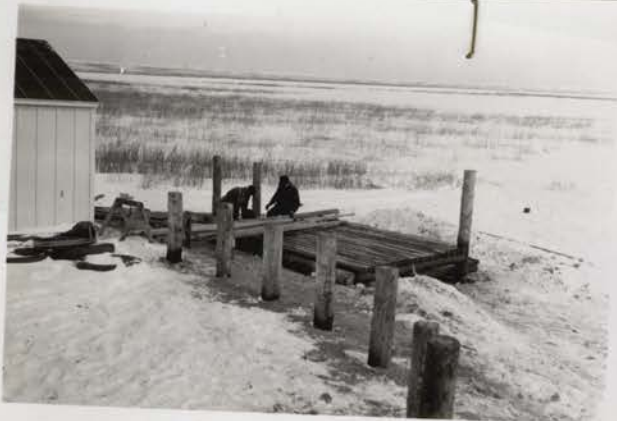
#555 Completed trail crossing (rip-rap*) below 50 control structure in old dike.
