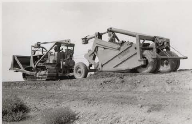
#561 Loading Letourneau in travel leveling operations on Dry Lake supply canal bank.
