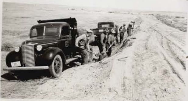
#559 Hand loading surplus fill in dry Lake supply canal bank for use in filling low placed in construction of trail on this bank.
