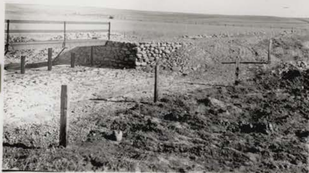
#555 Completed trail crossing (rip-rap*) below 50 control structure in old dike.
