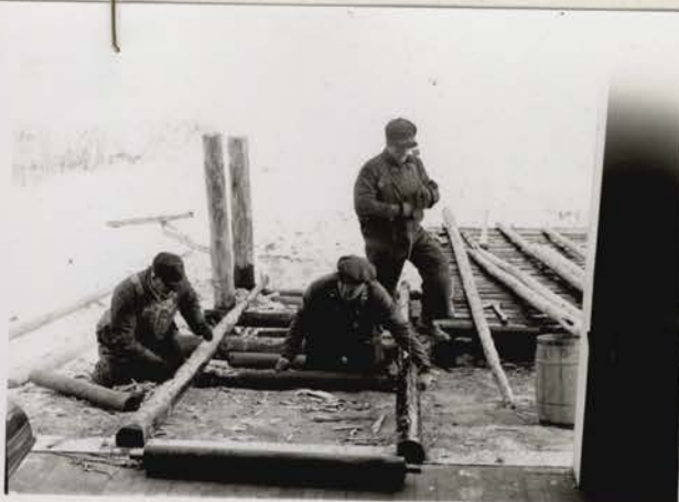
#556 Cat-walk and graveling top of wing-wall fills completed on 50 ft. structure in old dike. Town of Bowdoin in background
