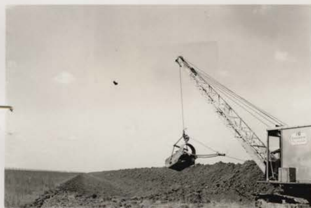
#565 Dragline excavating drain canal and casting dirt for fill in Dry Lake dike. Note uniformity of both fill and canal
