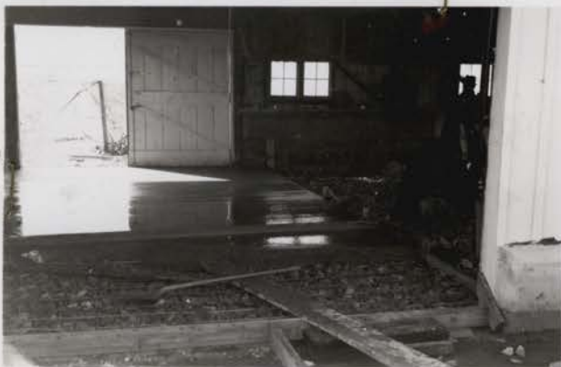
#563 Floating down a section of the steel reinforced concrete floor in equipment Bldg.
