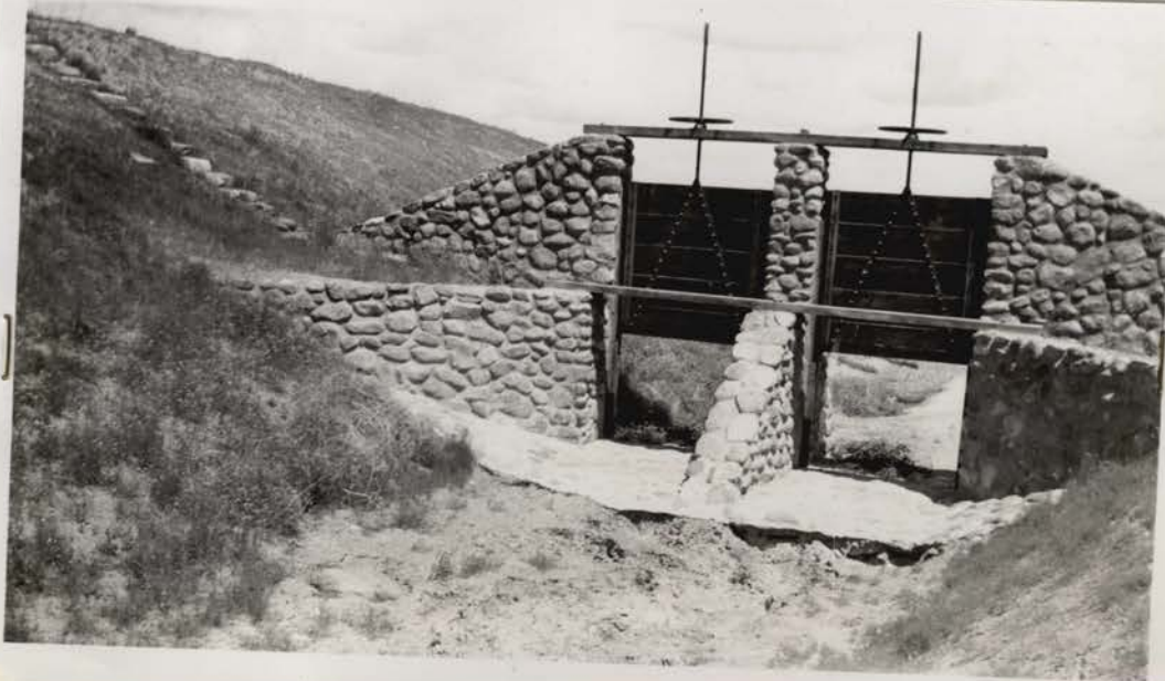
#571 Diversion canal outlet gates need some repair on lower side of masonry footings.
