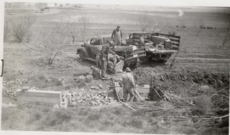
No. 751 7-15-43 Building trap to stop fish from leaving storage reservoir when irrigation water is taken out. State Fish and Game men doing work with our coop- eration.
