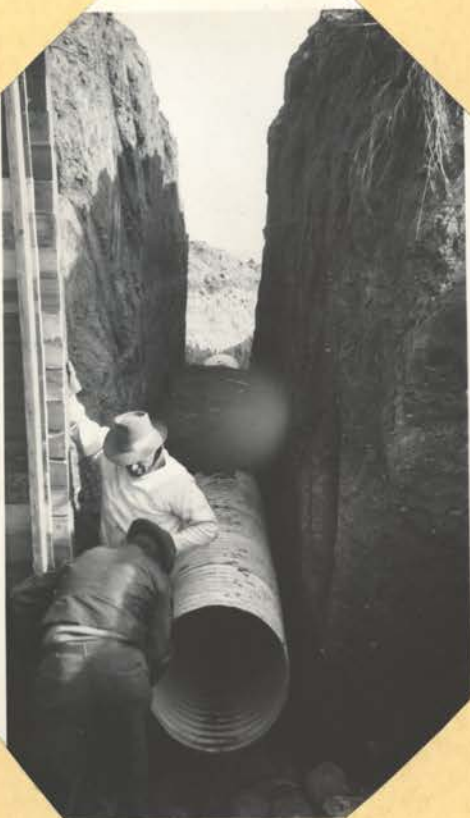
Upper R32 E-1 Apr. 30 Starting excavation on the new 500 ft. sewer line at hdq. Dragline is one that State Fish & Game had here for work on fish pond. Gravel on right is for the drain field. Lower R32 E 2&3 Apr. 4 & 5. Cut, Culvert and nearly completed forms on the new fish trap and spillway in the hdq irrigation reservoir. The reservoir is used cooperatively by the State Fish & Game Dept. as a rearing pond for Pike.
