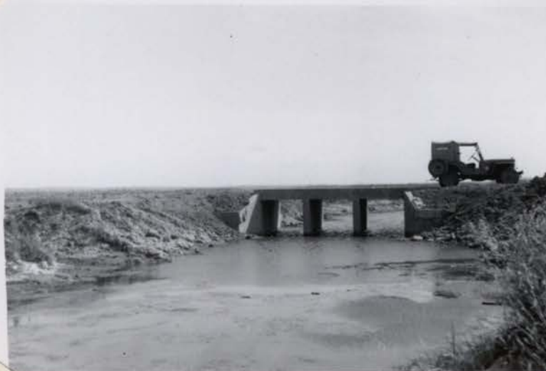
R-84, E-8 (8/10/53) Contract bridge #11 completed except for rip rap of wings and aprons.
