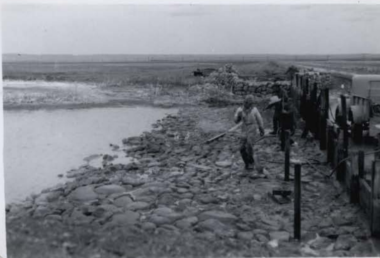
R-79, E-7 (5/12/53) Cleaning rubble base and cutting down flashboard steel structure in reversion of flashboard structure #2 to contain a bridge structure also.
