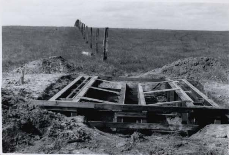
R-81, E-2 (6/5/53) Excavation and forms in place for installation of Lincoln steel gattle gates.
