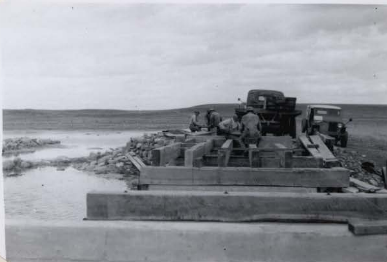
R-79, E-8 (5/14/53) Installation of pier caps, stringers and decking for bridge and flashboard structure #1.
