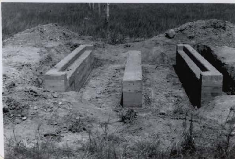
R-81, E-3 (6/18/53) Concrete has been poured and forms freshly stripped for installation of cattle gate.
