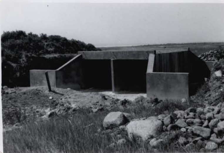
R-83, E-2 (7/12/53) Completed reinforced concrete bridge #10. Five of this type bridge were constructed by contract during this period.
