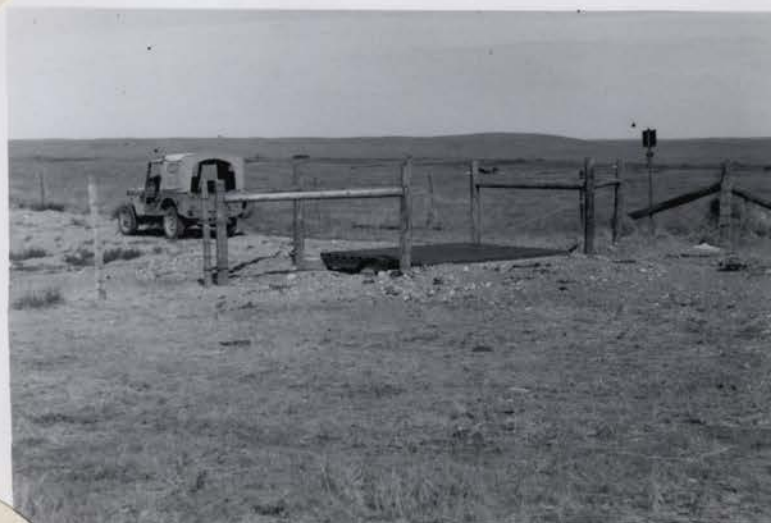
R-84, E- 2 (8/10/53) Complete installation showing tie in with fence lines. Six such cattle gates were installed at Bowdoin this period.
