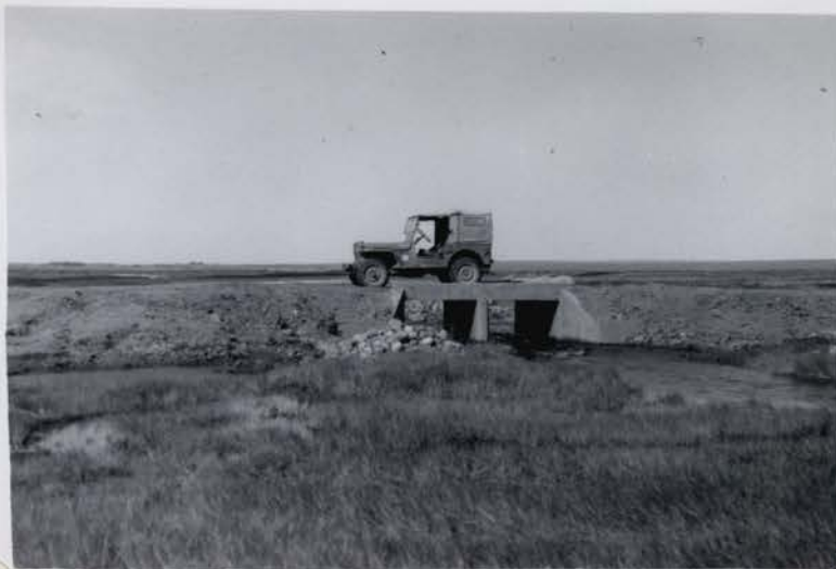
R-84, E-5 (8/10/53) Completed bridge #10 except for rip rap of wings and apron. Approx. 25 S.F. flow going through bridge to Lake Bowdoin.
