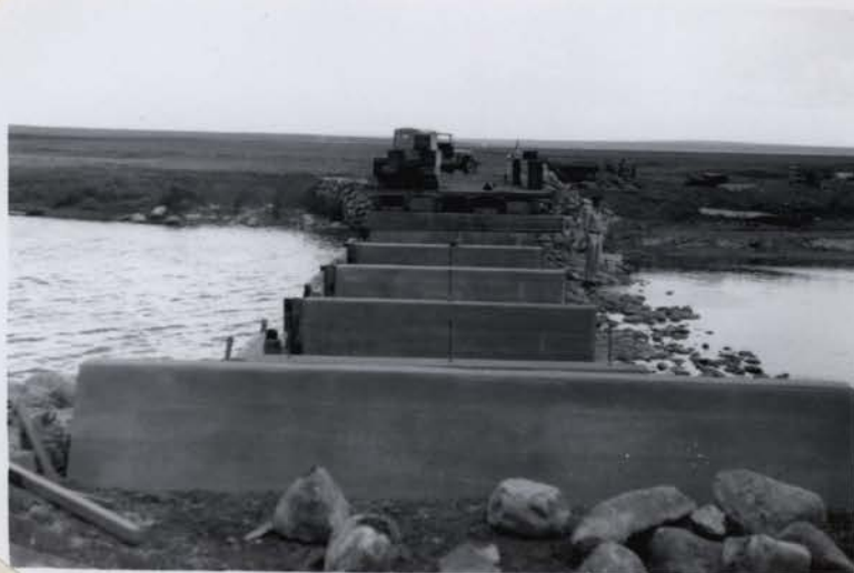
R-81, E-6 (6/20/53) Completed concrete work and start on installation of pier caps, stringers and decking of reconverted structure #2.
