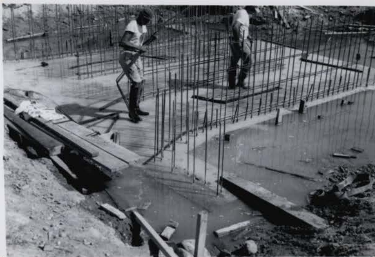
R-84, E-1 (7/21/53) Placing pier and abutment steel on contract bridge #11. Slab poured 7/20/53.
