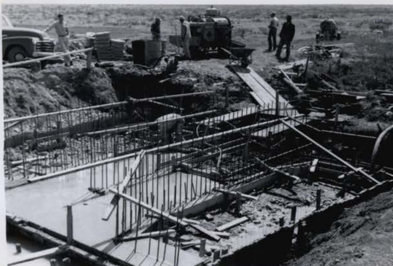
R-81, E-4 (6/20/53) Contract bridge crew pouring cutoff walls and floor slab for reinforced concrete bridge #10 at Bowdoin.
