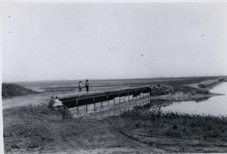
R-83, E-3 (7/12/53) Reconverted bridge and flashboard control structure #2 100% complete and ready for use. This along with structure #1 on east end of dike C insure year around access to dike C with any type of equipment.
