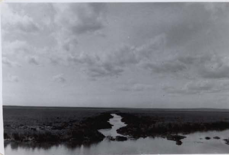
R-79, E-4 (4/22/53) This opening exclusive of the first charge shown above was all obtained by one blast. 400 lbs. of 40% ditching powder was used for the entire job.
