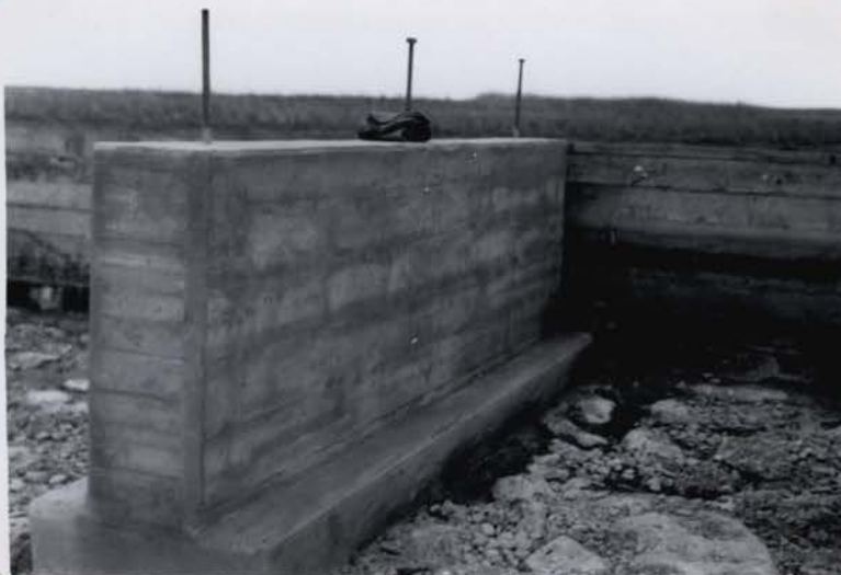
R-81, E-5 (6/20/53) One of 7 completed concrete piers of reconverted combination bridge and flashboard control structure #2.
