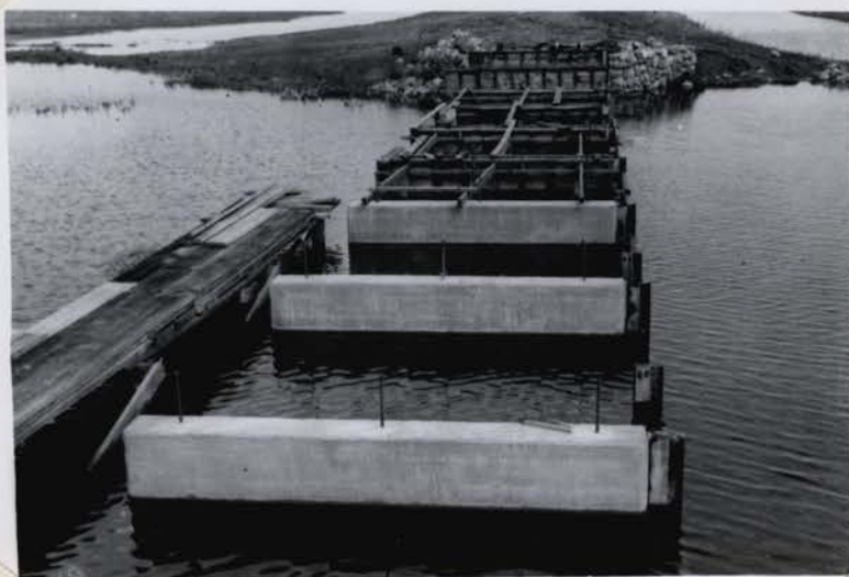
R-81, E-1 (6/5/53) May and June rains considerably hampered bridge construction work. Here about 3\frac{1}{2} feet of water over a sizeable area had to be pumped out with a 2 inch pump before construction could be continued.
