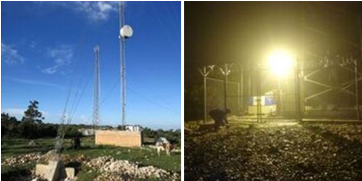
Figure 3.9. Communication towers near Black-capped Petrel nesting areas on Hispaniola. Height of structures and associated guy wires depicted in left image; nighttime security lights depicted in right image. A disoriented and grounded Black-capped Petrel also being recovered from the ground in right image. Photos by J. Goetz.
