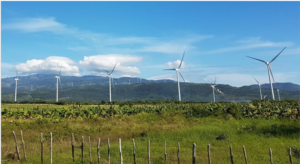
Figure 3.11. Inland wind farm in the southwestern Dominican Republic and located between the coastline and a Black-capped petrel nesting area of Loma Quemada, Sierra de Bahoruco. Note presence of wind turbines also on a ridge in the background. Photo by A. Jhonson-Camacho, January 2018.
