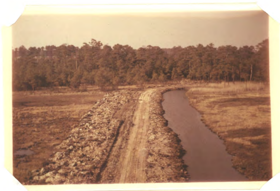
Photo #12. Same road after widening by use of Dragline. #42-459
