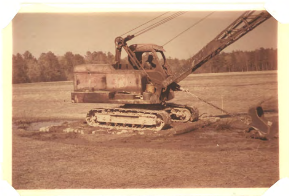
Photo #10. Dragline used in ditching under APW Project. Forced to use matts due to wet conditions. #42-457
