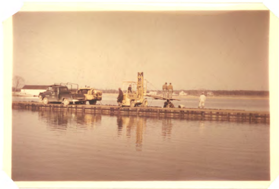
Photo #5. Installing Wakefield piling on Headquarters Dike Road under APW Project. #42-452
