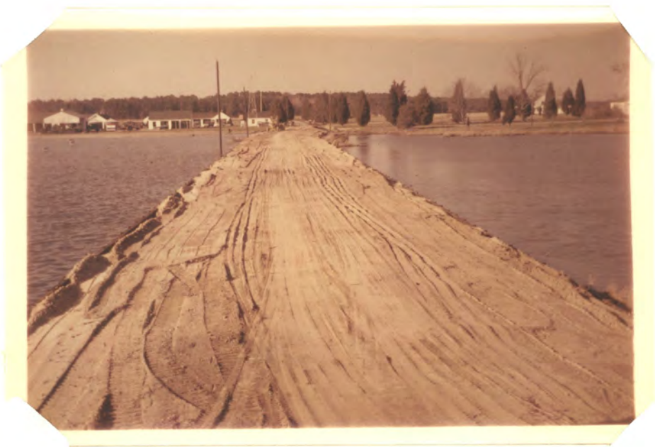
Photo #6. Road after Wakefield installed and fill placed on same. #42-453
