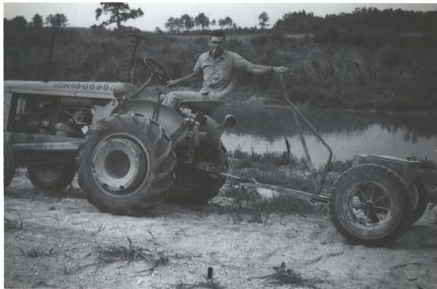
Photo. #20 Spreader used in applying soil amendments and seeding of new dike bank slopes. #42-617
