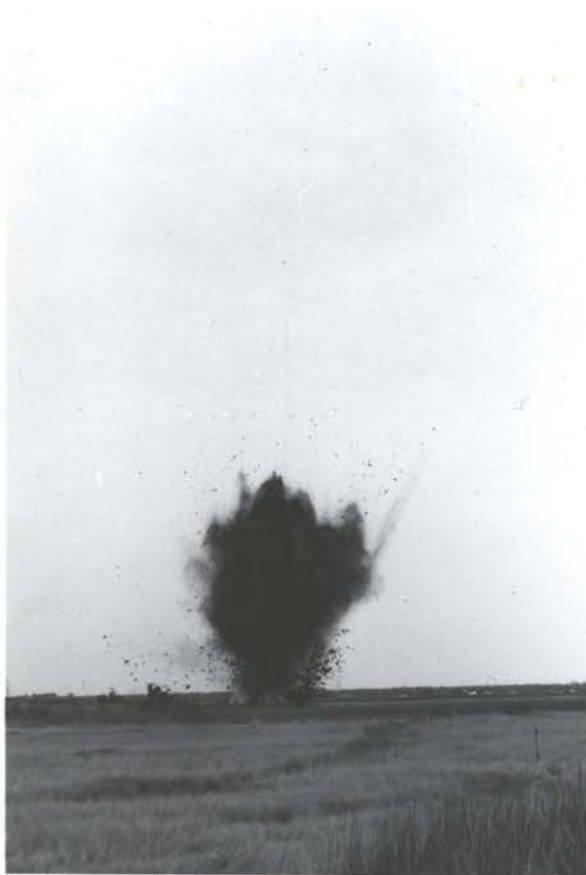
Photo. #104- Pot-hole blasting with ammonium nitrate and diesel fuel mixture, triggered with dynamite. #42-772
