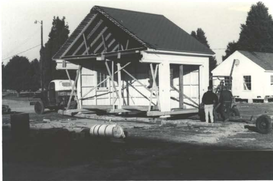
Photo #27. Three refuge buildings were declared excess and removed by local bidders. This building had to be cut in two before removal.
