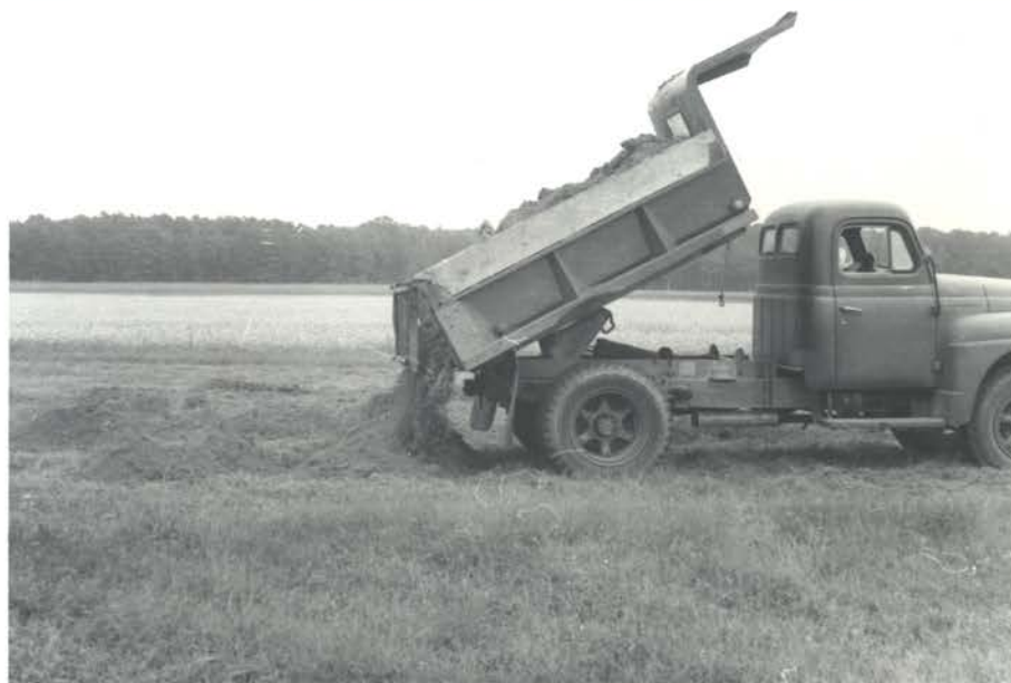
Photo #24. A new cannon net sight is being constructed at the Dieffenbach Pool area. A slightly elevated area was needed and thus fill was hauled in.
