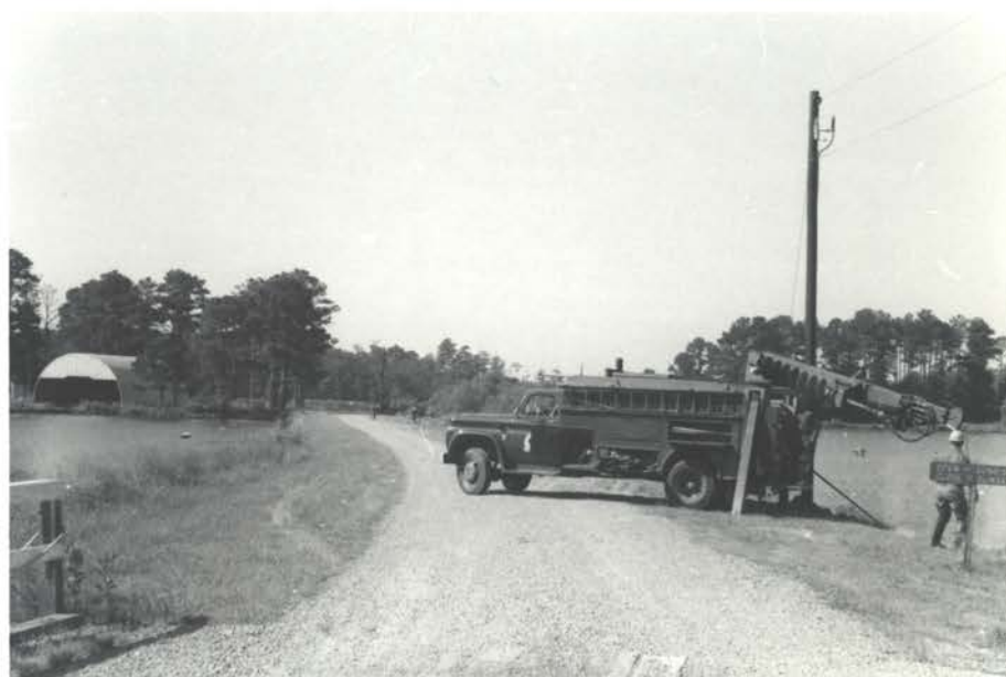
Photo #28. The power line leading across the Headquarters Pool dike was installed underground. This was done as a safety factor for the Management & Enforcement float plane.
